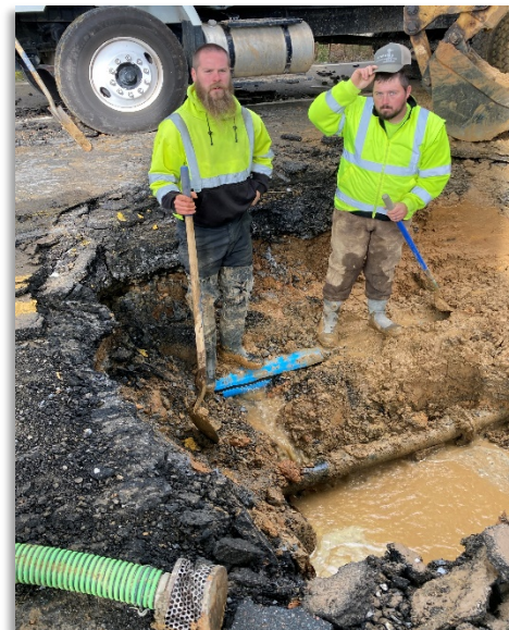
Main water line repair near Powder Branch and Milligan Highway.
