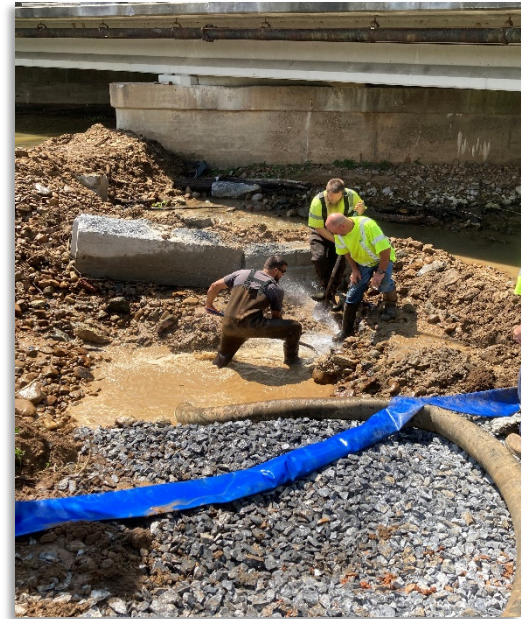
4" main line repair at Powder Branch and Milligan Highway.
