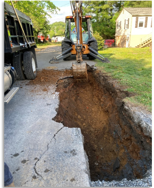
Preparing to install a manhole and new main line on Riverside.
