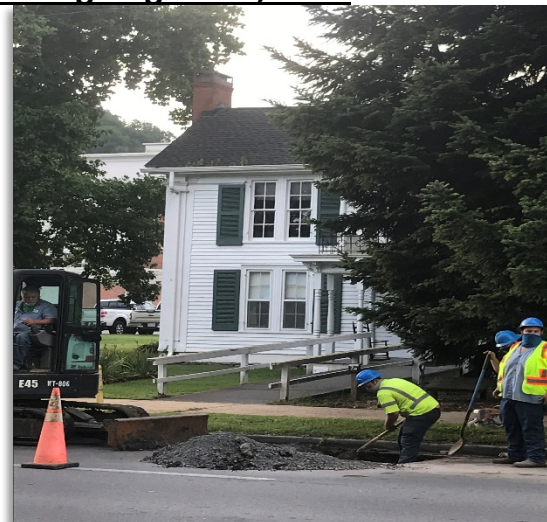
Crews complete a water line repair near the County Extension Office.
