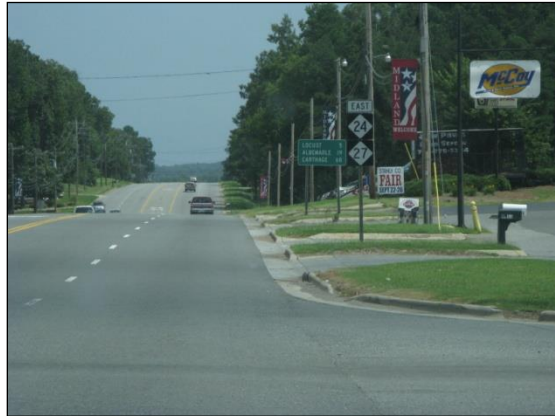
Intersection of NC Highway 24/27 and US Highway 601
