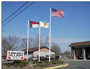
Midland Fire Station #1
