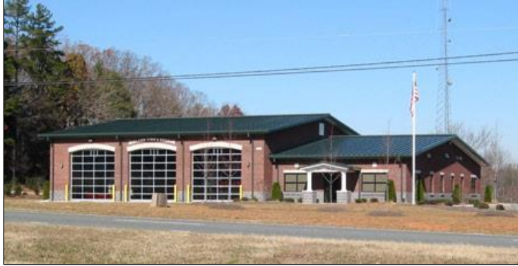
Midland Fire Station #2
