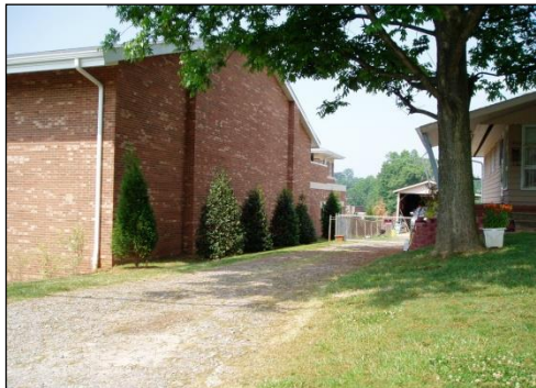
Inadequate Screening Between Uses
