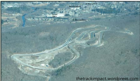
The track under construction, May 2015
