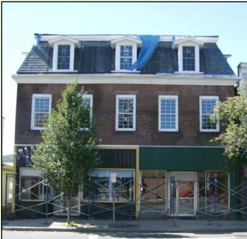
These photographs illustrate some of the challenges in Ware's downtown: vacant lots which leave holes in the streetscape, chronically vacant buildings, and uninhabitable buildings.
