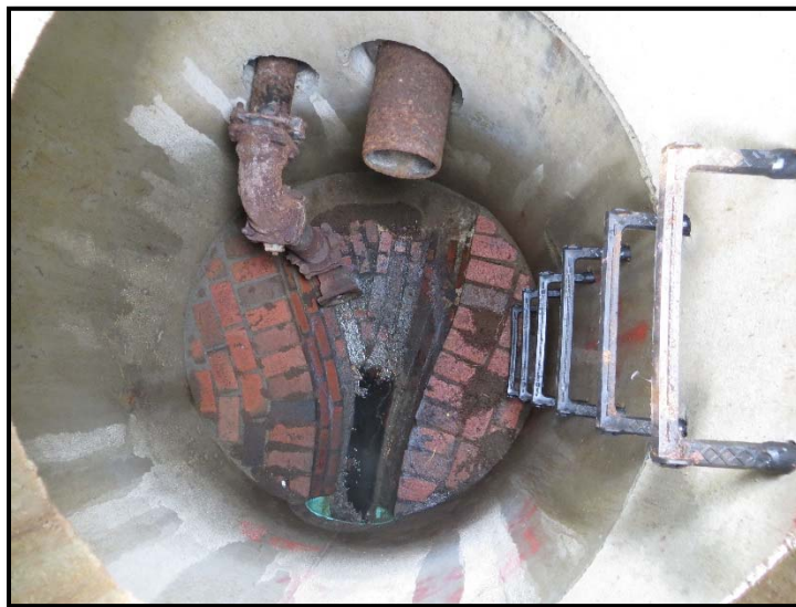
FIGURE 2-6 GIBBS CROSSING PUMPING STATION DISCHARGE MANHOLE
