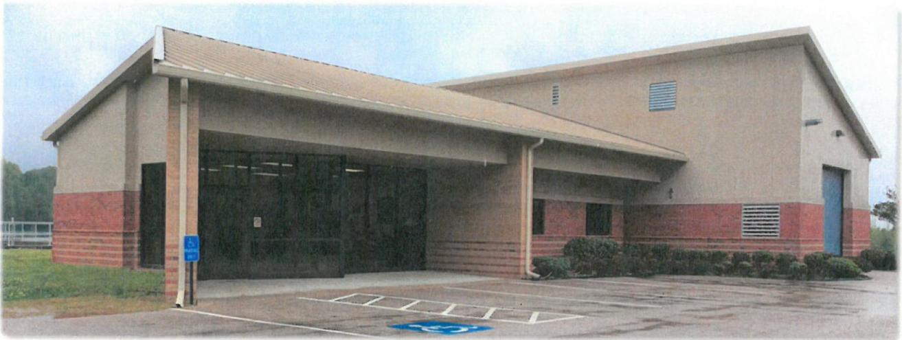
Arlington Wastewater Treatment Plant 11150 Highway 70
