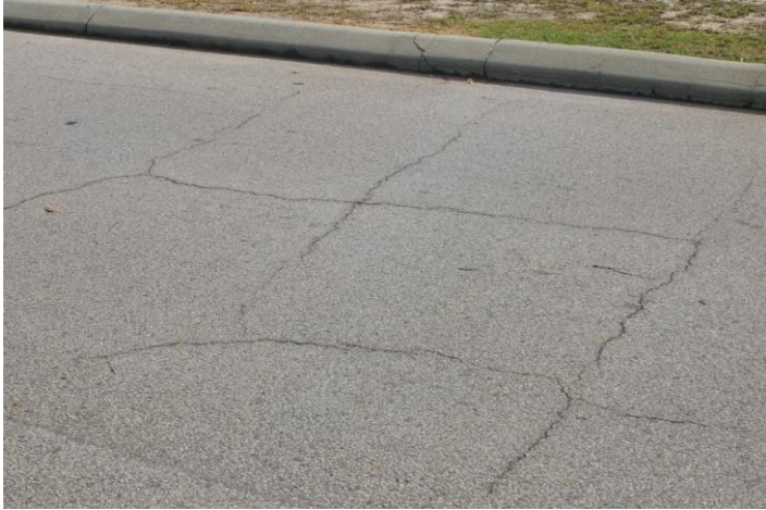
Block Cracking
