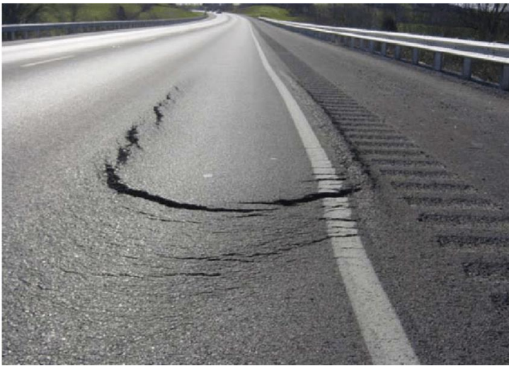
Slippage Cracking
