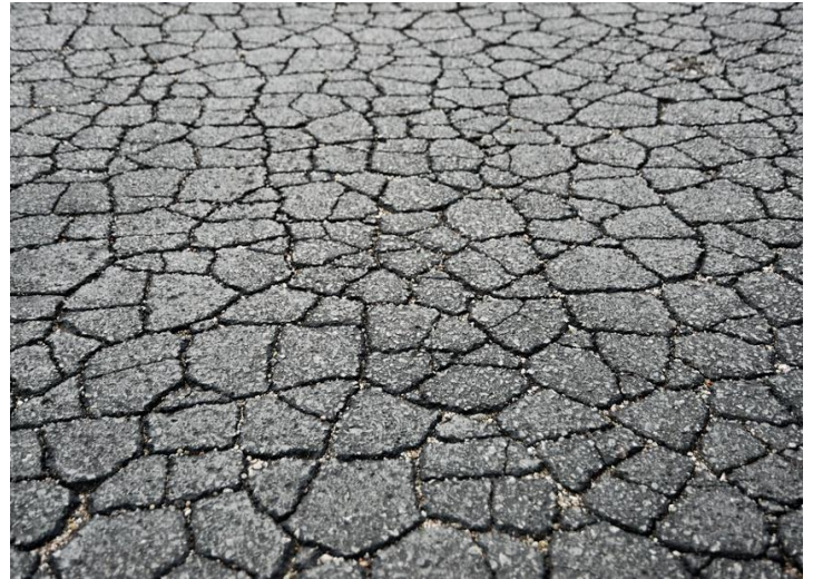
Alligator Cracking
