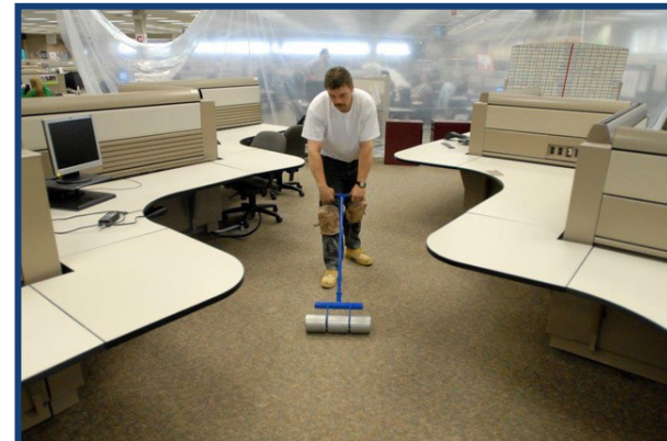
Roll the new carpet to ensure adhesion, and we are done!
