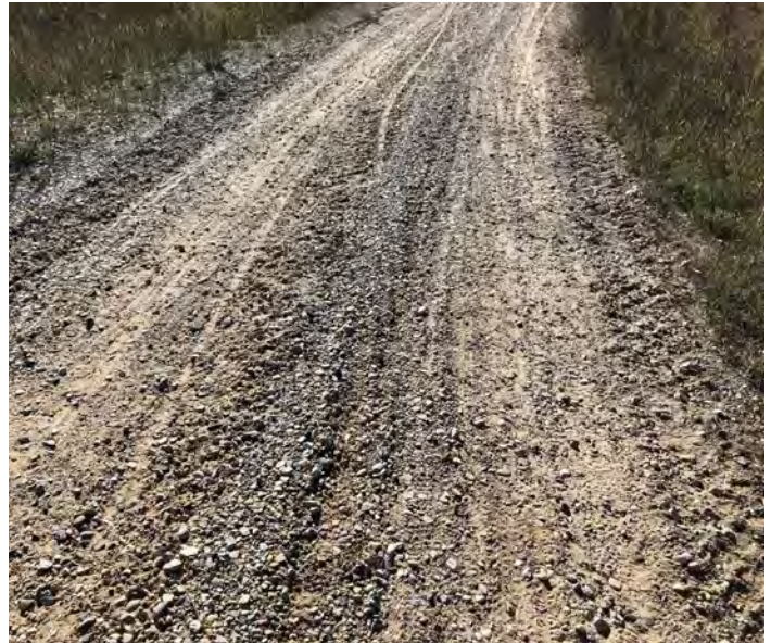
Example of loose, large aggregate gravel mix used for trail surfacing
