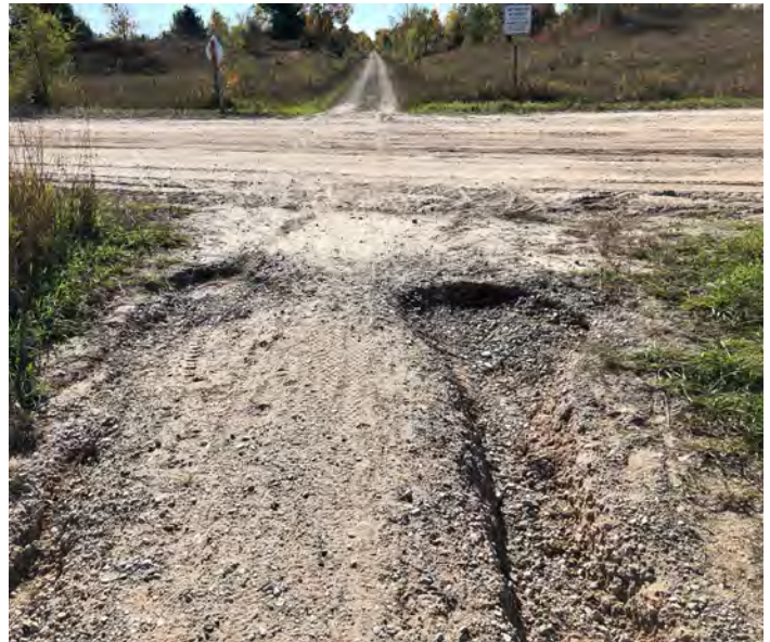
Erosion at the Gallagher Road crossing
