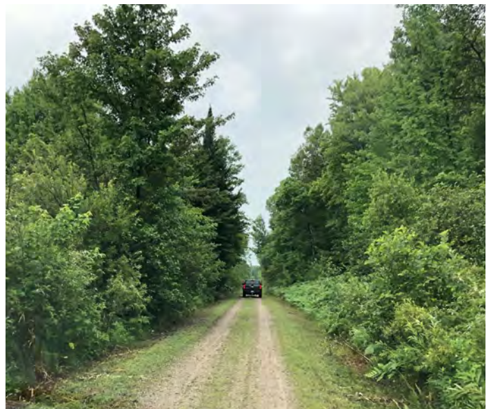
Vegetation growth in trail surfacing
