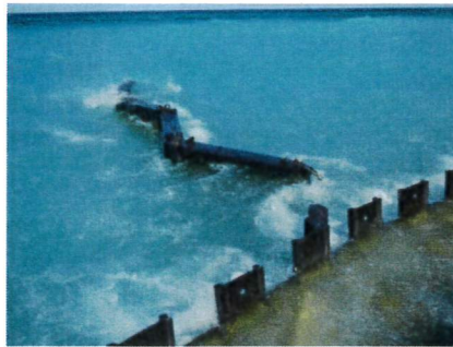
Figure 2.27: Groin 6 (looking west). Separation and bent or missing sheet between wall and groin.
