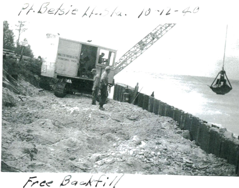
Figure 2.6: Construction of 1940-era SPS at Point Betsie, October 1940
