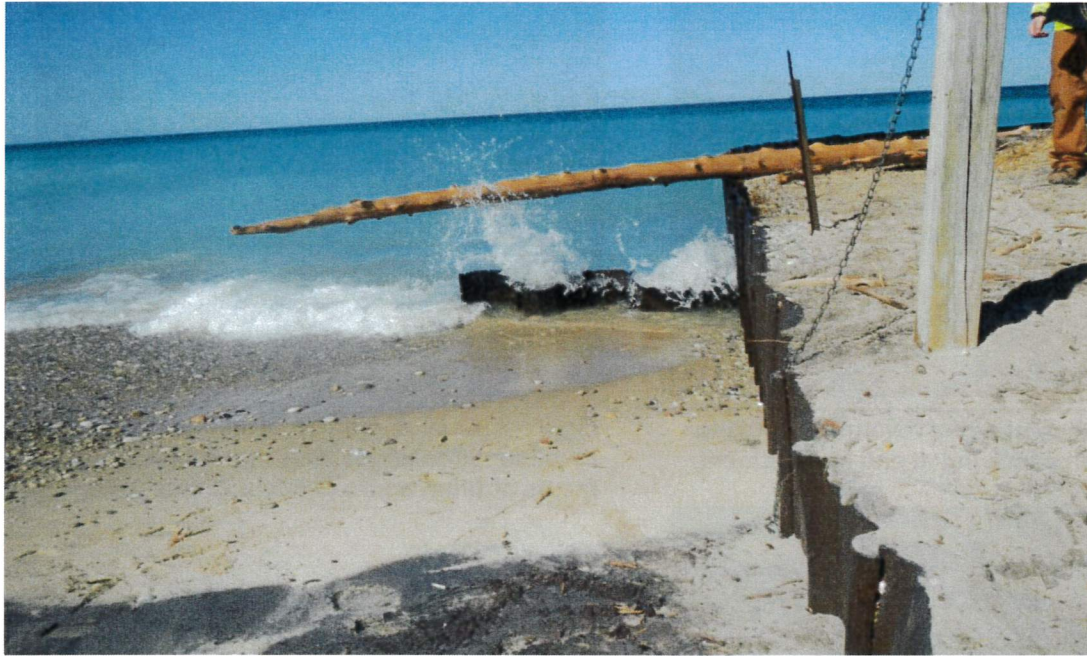
Figure 2.22: South return wall (looking west). Small lean in wall. Short curtain wall observed stemming out from south return wall.
