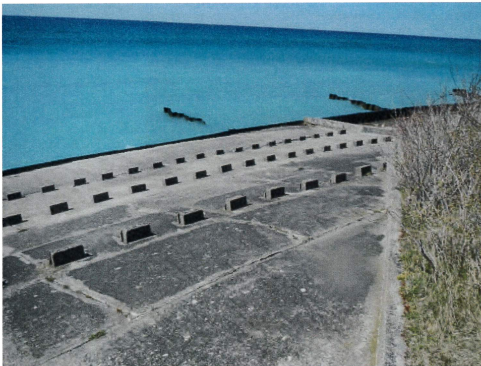
Figure 18: North concrete apron (looking northwest). Note difference in concrete coloration between lower apron and upper apron, as well as the different type of cinder block bollard (no flare on ends of newer cinder blocks, flat face).
