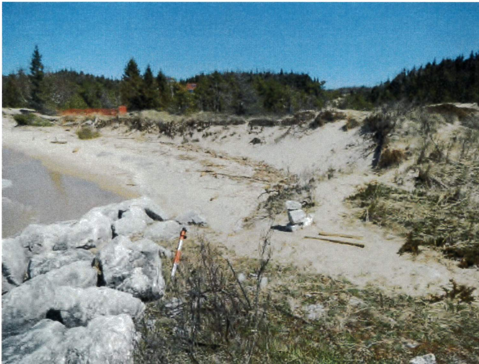
Figure 45: End of stone revetment (looking east). Erosion occurring at end of revetment.
