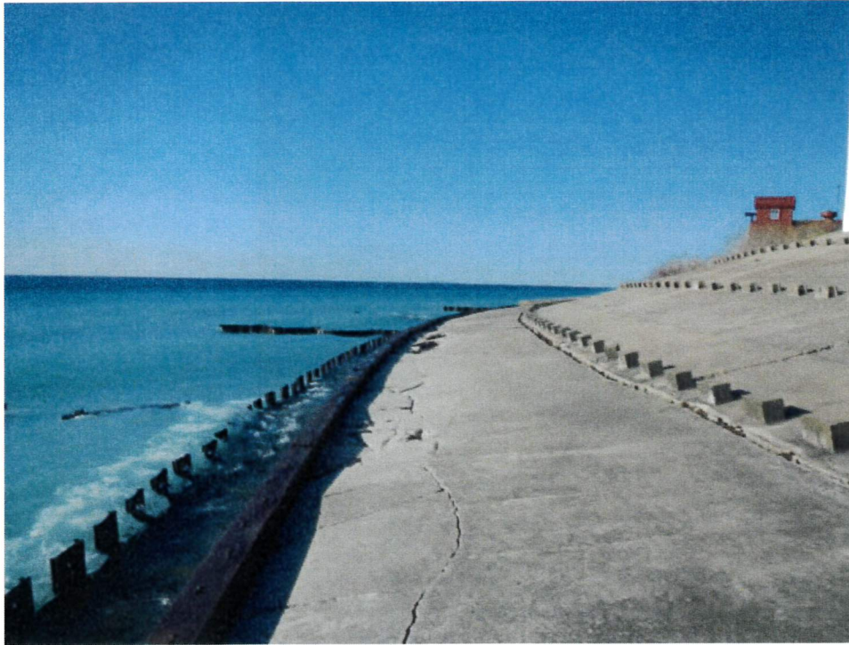
Figure 13: Concrete apron (looking north, just past the center point of the apron). Settlement and cracking.
