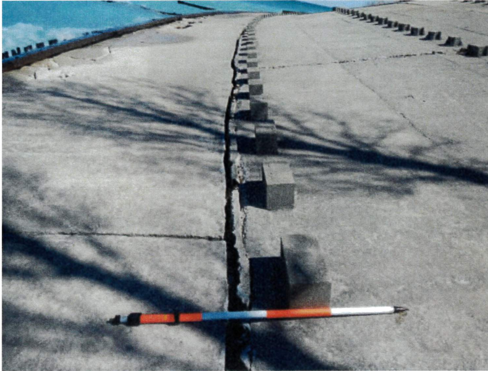
Figure 9: Concrete Apron (looking north, near center of apron). Separation of lower 13 feet segment of concrete apron. Note change in concrete coloration approx. 6 feet landward of lower apron separation.
