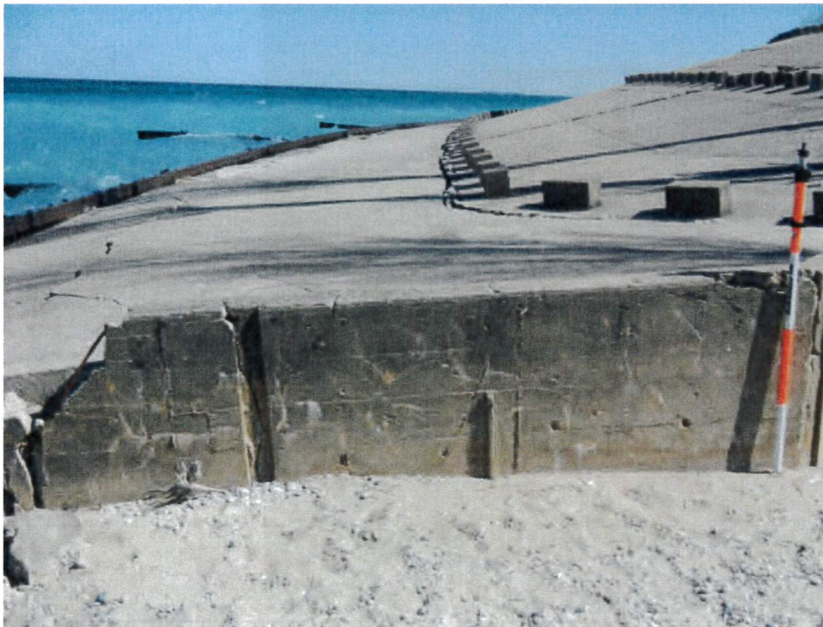
Figure 4: South Concrete Apron (Looking North). Concrete cracking within apron footing, mild efflorescence spider webbing.
