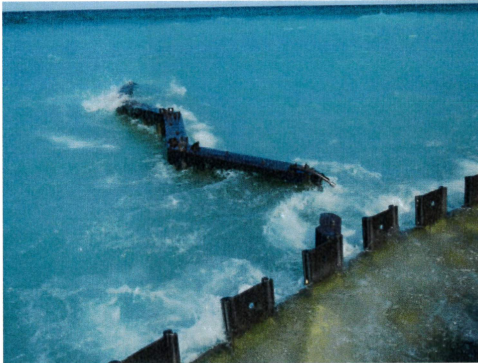
Figure 34: Groin 6 (looking west). Separation and bent or missing sheet between wall and groin.
