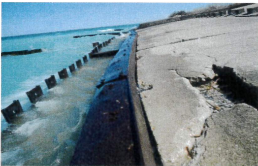
Figure 2.15: Steel cap beam and double wall (looking north, north apron curb can be observed). Distortion in steel cap beam, lean in wall. Cracking and spalling of apron.
