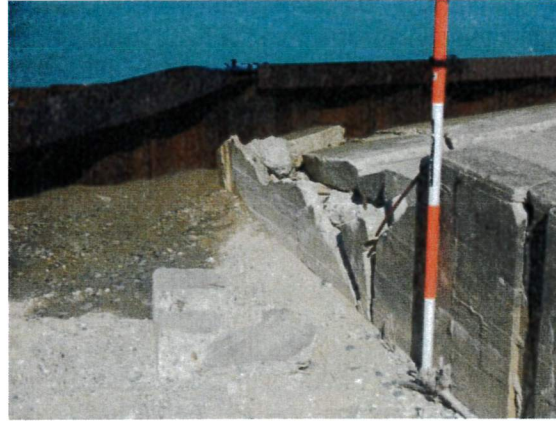
Figure 2.24: South Concrete Apron (Looking West-Northwest). Apron curb has cracked and settled. Some erosion and washout appears to have occurred to the south of the apron (once the concrete apron ends, extending all along the south extent to the South Return Wall).
