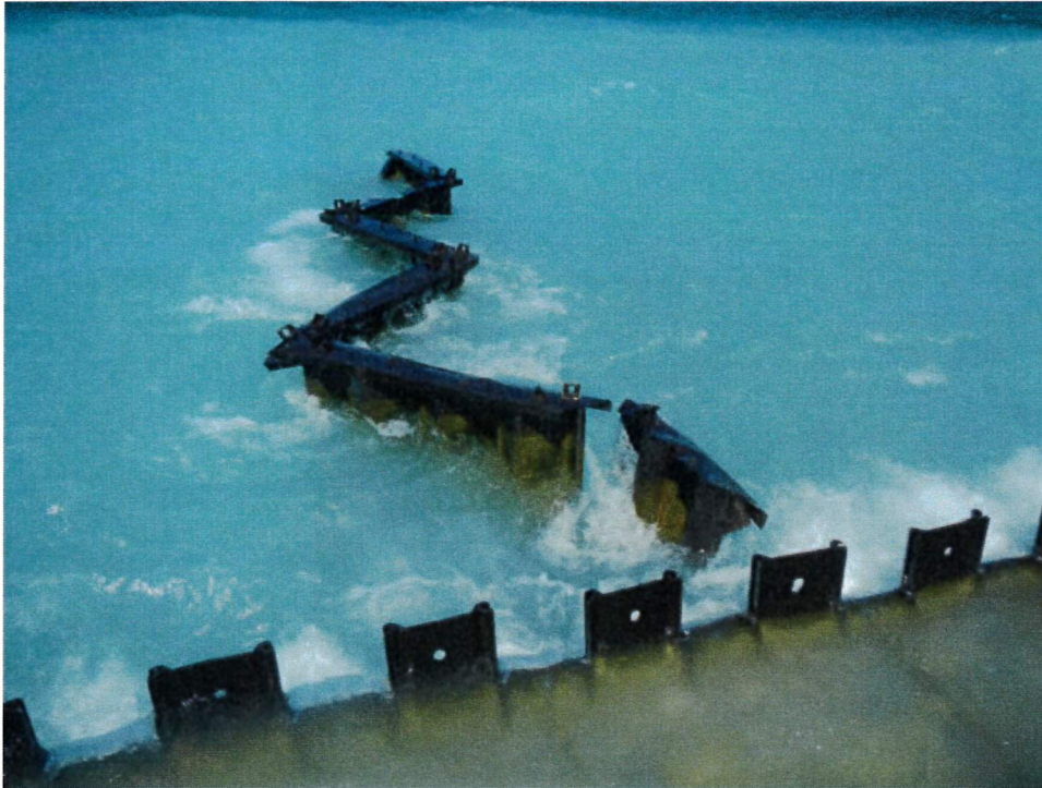
Figure 36: Groin 4 (looking west). Groin has separated from wall. First sheet pile pairs have lost interlock and are bent.
