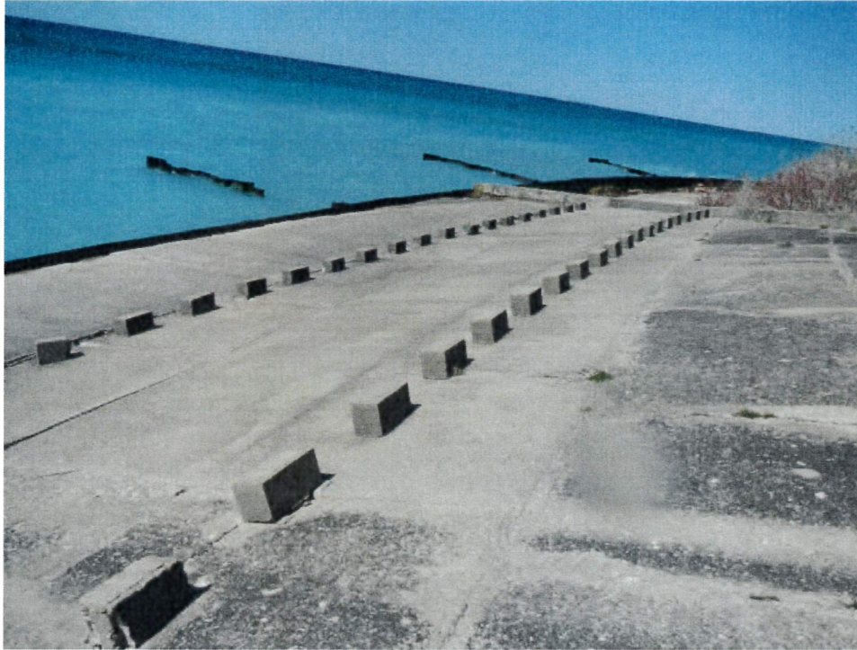
Figure 19: Lower portion of north concrete apron (looking north). Note difference in concrete coloration between lower apron and upper apron.
