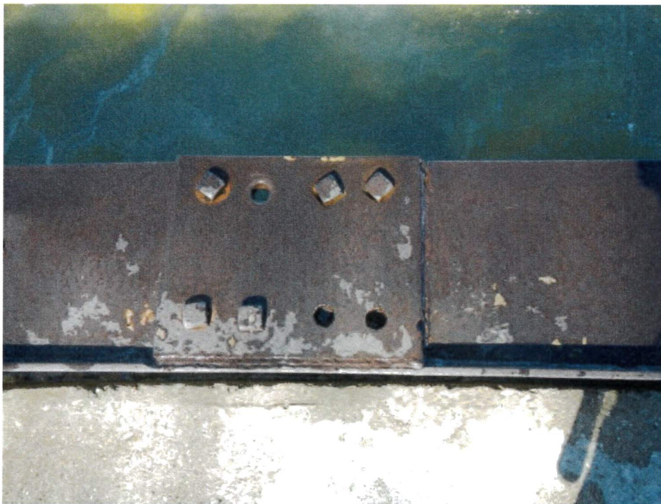
Figure 25: Typical missing and loose bolts at steel cap beam connection to bulkhead. Waves were observed to cause “clanging” in the cap beam due to it being loose.
