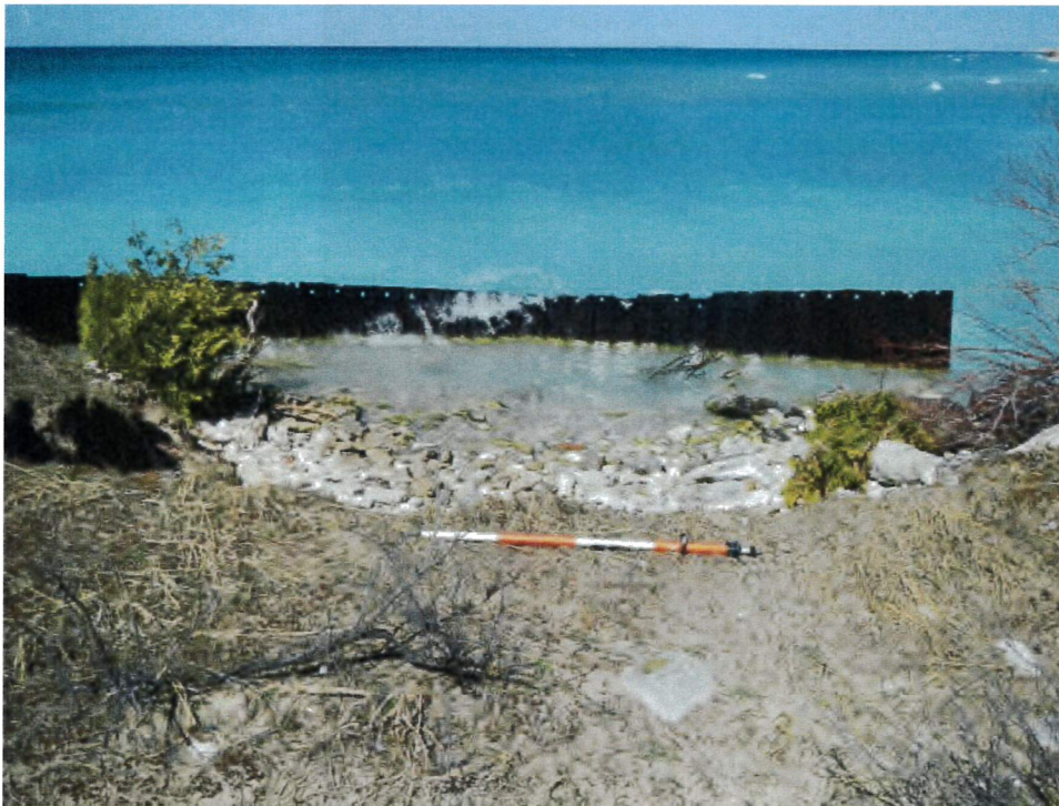
Figure 49: Bluff erosion at west end of stone revetment (looking north). Slope stability failure of bluff, approximately 25 feet wide.
