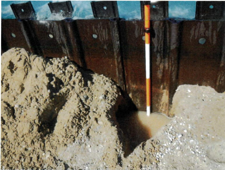
Figure 24: Hole dug on landward side of landward steel sheet pile at known tie rod location. Tie rod did not penetrate wall, indicates tie rod may have been welded to the waterside face of the sheet pile.
