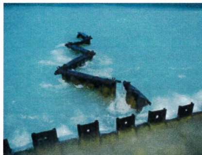
Figure 2.29: Groin 4 (looking west). Groin has separated from wall. First sheet pile pairs have lost interlock and are bent.
