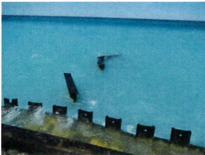
Figure 2.28: Groin 5 (looking west). Separation between wall and groin. Two areas where sheeting appears to be missing
