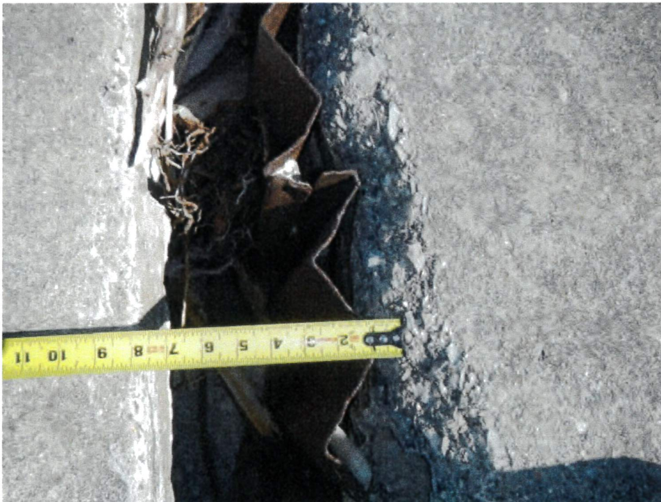
Figure 10: Close view of separation between lower 13 feet segment of apron and the upper portion of apron.
