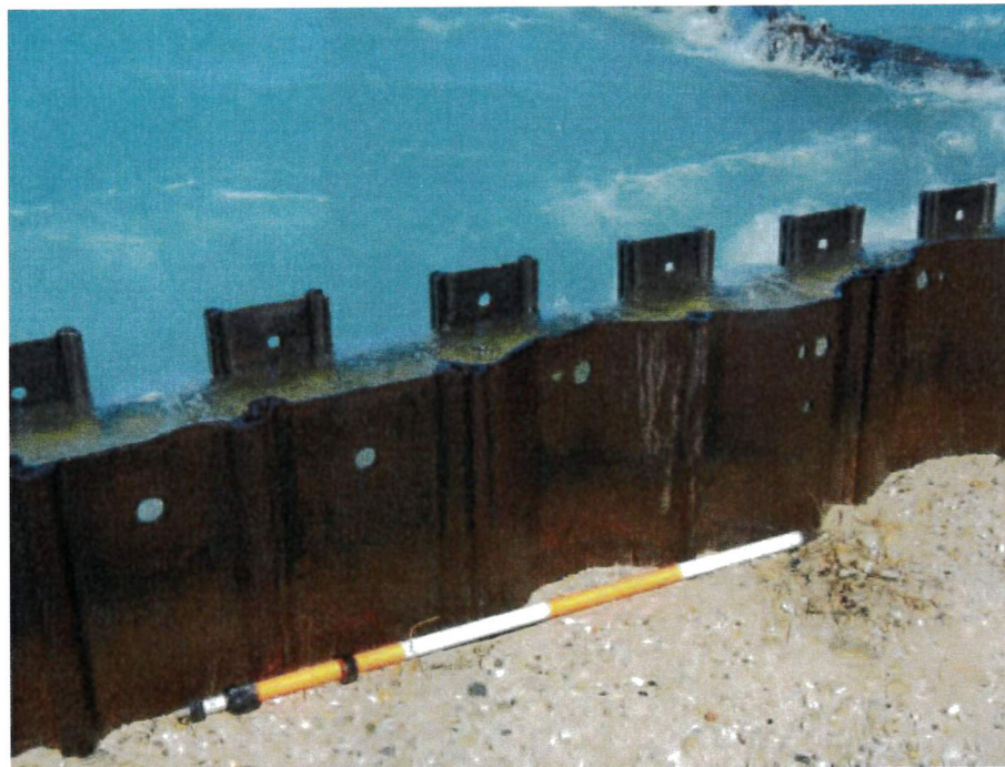
Figure 23: Transition in landward sheet pile wall to from “straight” sheets to “z-sheets” (looking west, to the south of the concrete apron).
