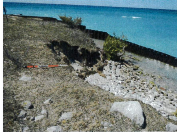
Figure 2.20: Bluff erosion at west end of stone revetment (looking northwest). Slope stability failure of bluff, approximately 25 feet wide.
