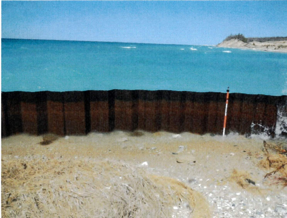
Figure 54: Erosion behind north return wall (looking north).
