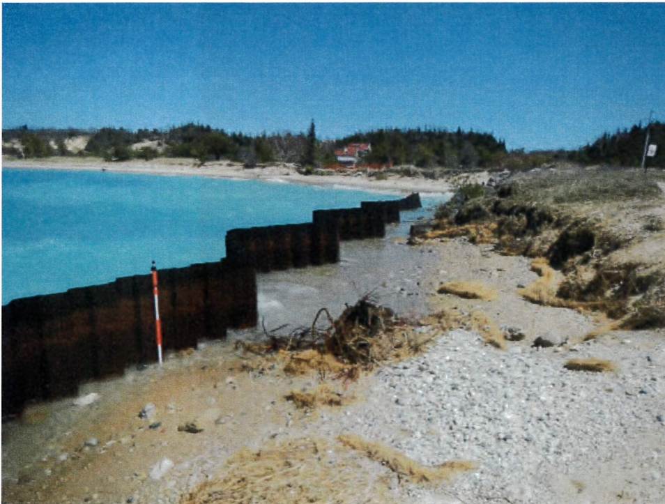
Figure 53: Erosion behind north return wall (looking east). Erosion extends 20 to 30 feet behind sheet pile return wall.
