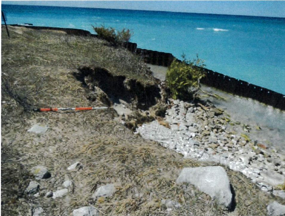
Figure 52: Bluff erosion at west end of stone revetment (looking northwest). Slope stability failure of bluff, approximately 25 feet wide.
