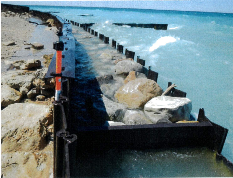
Figure 30: Channel cross-beam near termination of steel cap beam (looking south, north end of apron can be seen). Note the erosion that has occurred behind the double sheet pile wall.
