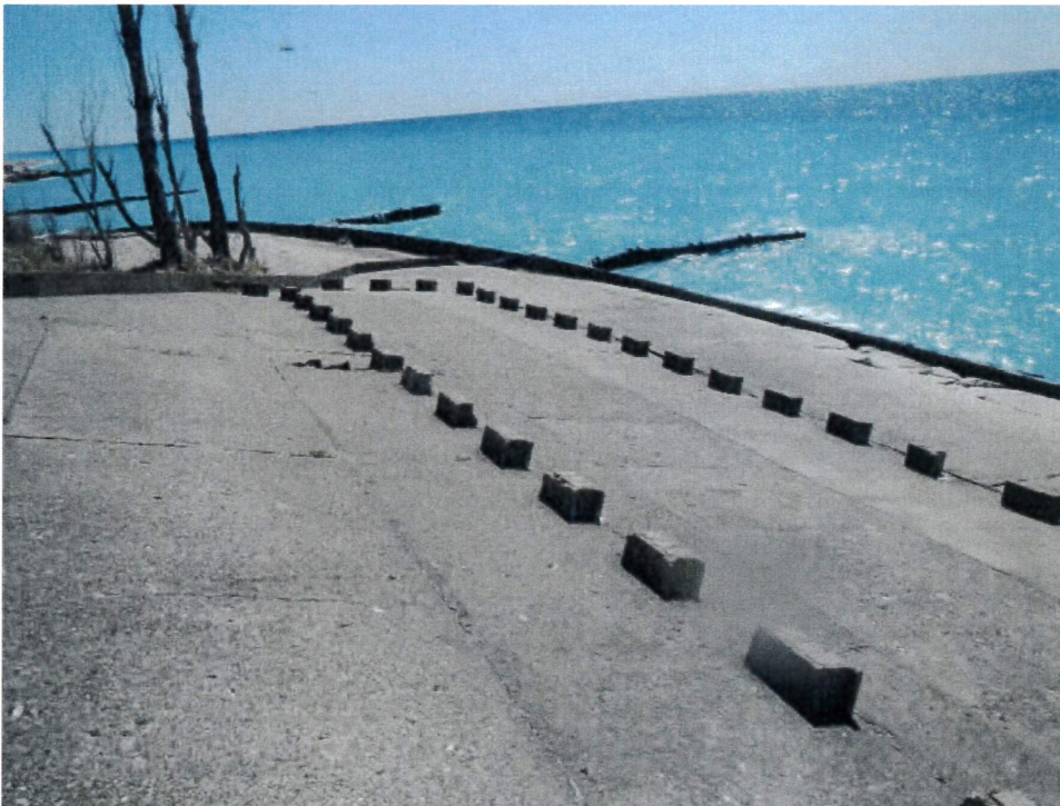
Figure 20: Lower portion of south concrete apron (looking south). Note difference in concrete coloration between lower apron and upper apron.
