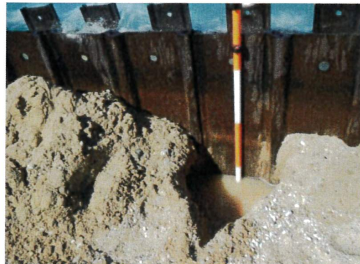
Figure 2.15: Hole dug on landward side of landward steel sheet pile at known tie rod location. Tie rod did not penetrate wall, indicates tie rod may have been welded to the waterside face of the sheet pile.
