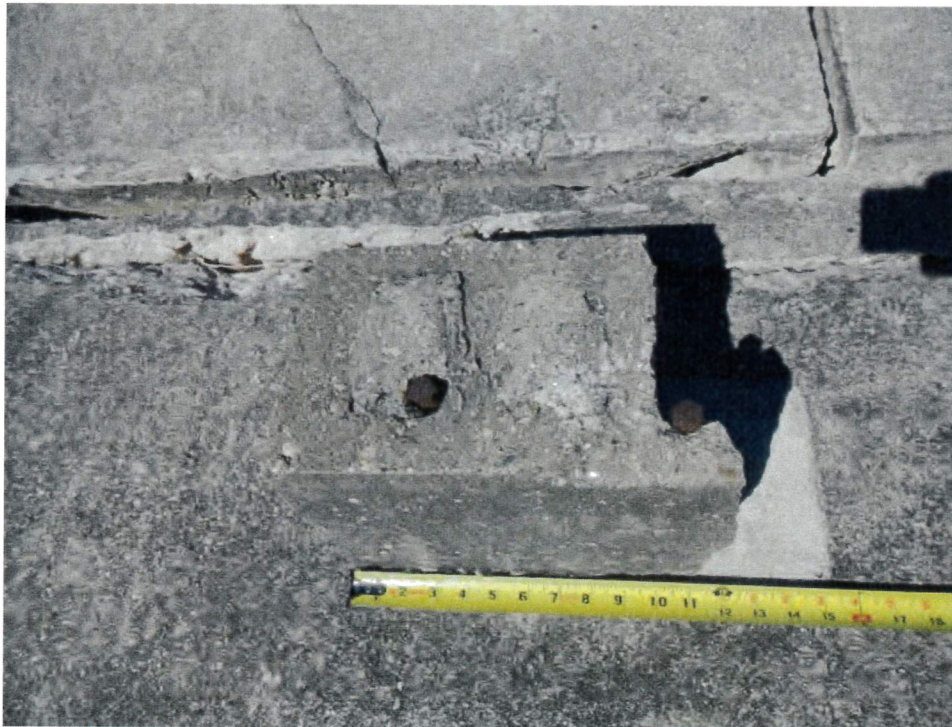
Figure 12: Typical cinder block bollard. Note rebar dowels can be observed.
