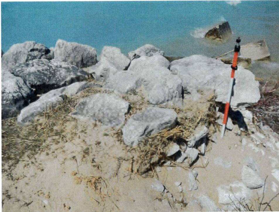
Figure 46: End of stone revetment (looking north). Erosion occurring at end of revetment.
