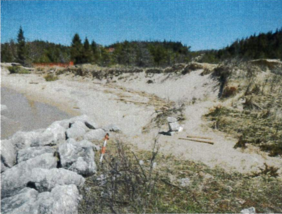
Figure 2.19: End of stone revetment (looking east). Erosion occurring at end of revetment.
