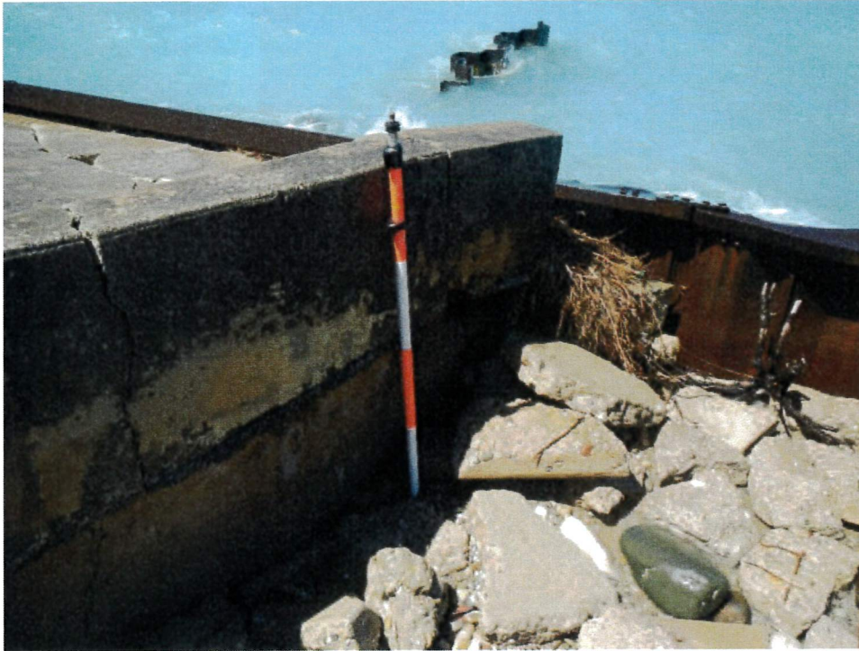
Figure 17: North concrete apron (looking southwest). Minimum of 2 feet erosion, exposing lower portion of original footing. Debris collection. Cracking in apron footing.
