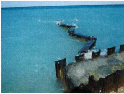
Figure 2.26: Groin 7 (looking west). Separation observed between wall and groin
