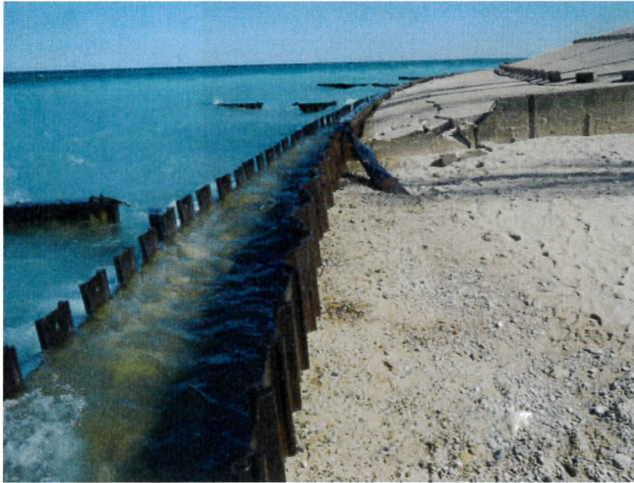
Figure 3: South Concrete Apron (Looking North). Steel channel has been damaged. Apron has severed from the steel sheet pile, settled in the order of 12 to 18 inches, significant cracking. Double sheet pile wall is leaning 4-6 inches.
