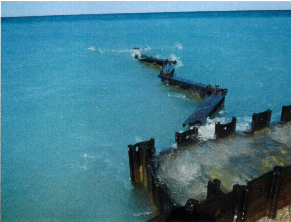
Figure 33: Groin 7 (looking west). Separation observed between wall and groin.
