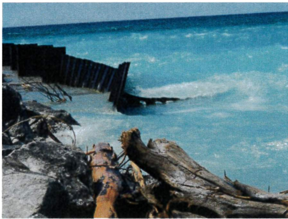
Figure 2.16: End of north wall return (looking west). Severe wall lean. Loss of interlock and sheet pile bending.
