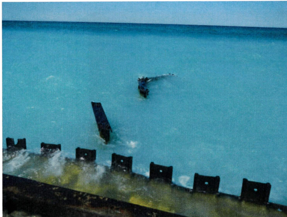
Figure 35: Groin 5 (looking west). Separation between wall and groin. Two areas where sheeting appears to be missing.
