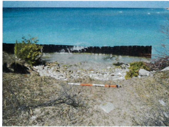
Figure 2.17: Bluff erosion at west end of stone revetment (looking north). Slope stability failure of bluff, approximately 25 feet wide.
