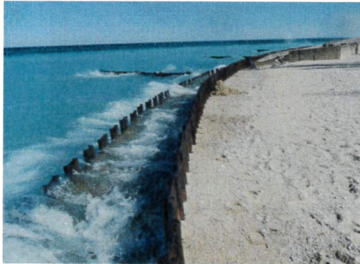
Figure 2.15: Typical lean in double sheet pile wall (looking north, to the south of the concrete apron). Lean in wall ranged from 4 to in excess of 6 inches.
