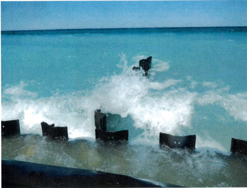
Figure 38: Groin 2 (looking west). Separation between wall and groin. Several sheet piles appear to be bent or missing.
