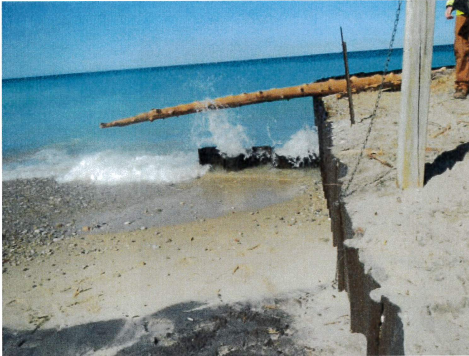
Figure 42: South return wall (looking west). Small lean in wall. Short curtain wall observed stemming out from south return wall.
