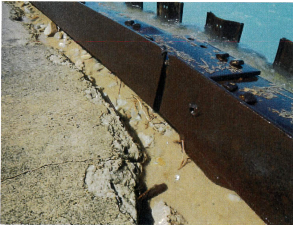
Figure 16: Typical apron dowel location. Dowel welded to steel cap beam has severed (at all locations along length of apron).
