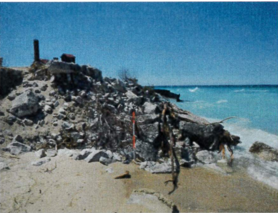
Figure 2.21: End of stone revetment at north return wall (looking west). Erosion. Sever wall lean.
