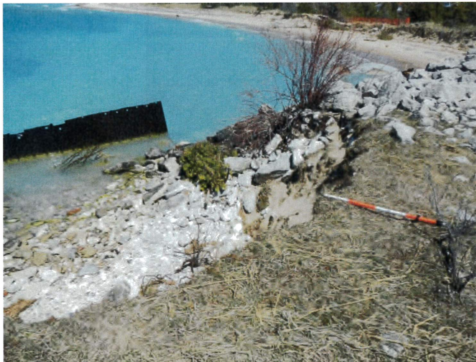
Figure 51: Bluff erosion at west end of stone revetment (looking northeast). Slope stability failure of bluff, approximately 25 feet wide.
