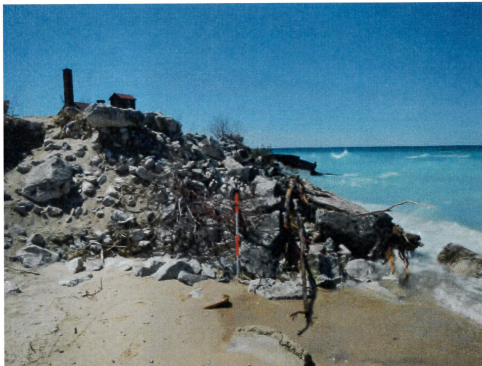
Figure 47: End of stone revetment at north return wall (looking west). Erosion. Sever wall lean.
