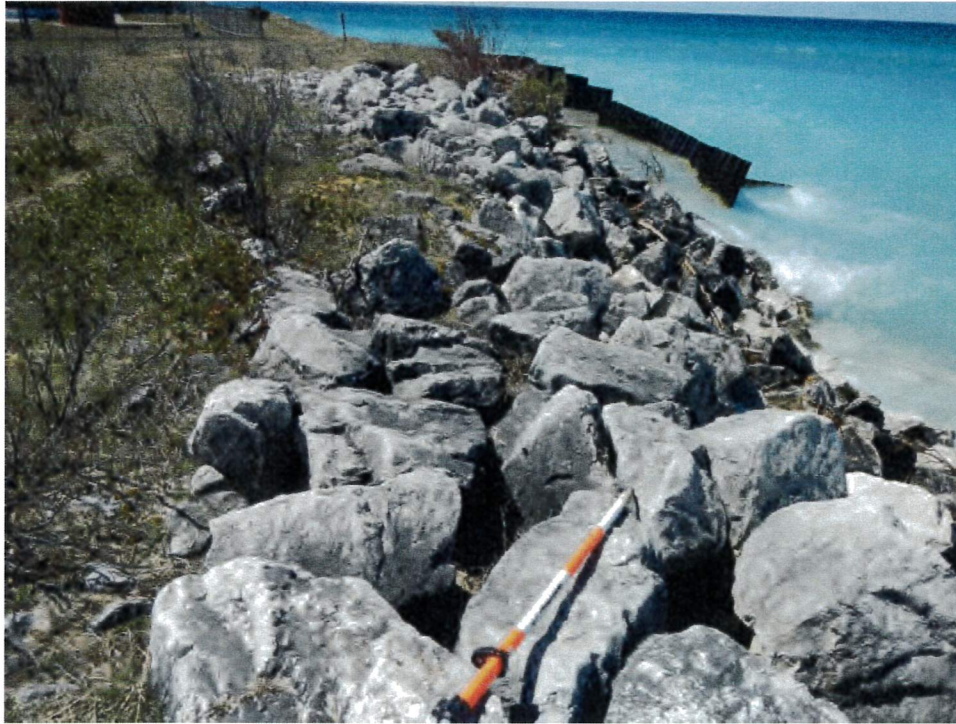
Figure 44: North return wall (looking west) at end of stone revetment. Erosion and severe wall lean.
