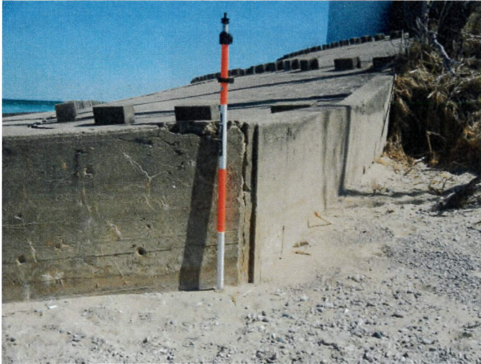
Figure 5: South Concrete Apron (Looking Northeast). Cracking and separation of lower apron from upper apron. Lower apron is approximately 13' wide, from landward sheet pile to separation point.
