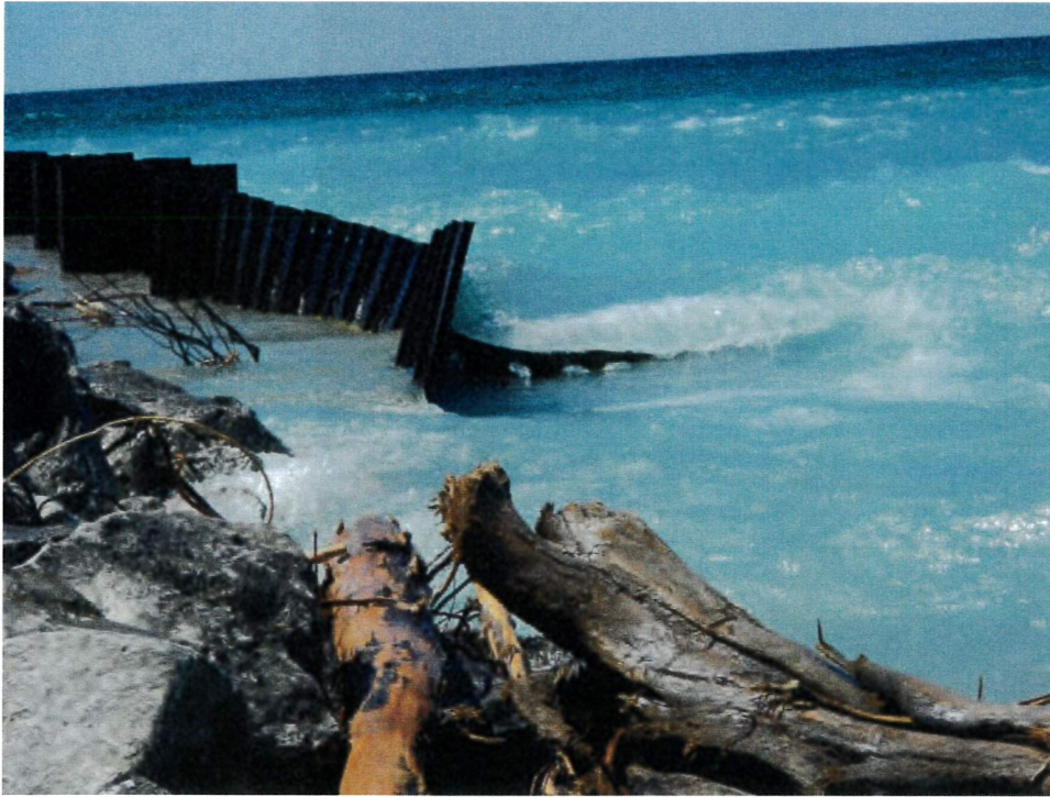
Figure 48: End of north wall return (looking west). Severe wall lean. Loss of interlock and sheet pile bending.
