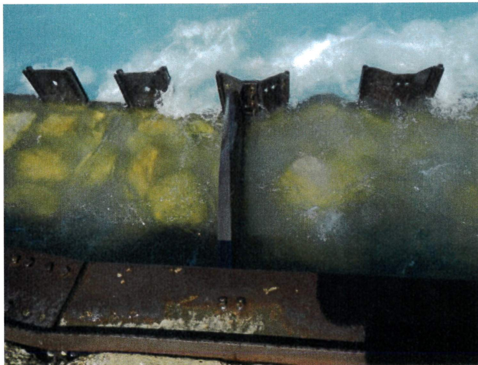
Figure 27: Distortion in steel cross-channel between double wall.
