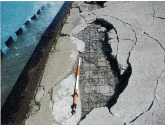
Figure 2.25: Concrete apron (close up of large cracking and spalled area). Exposed welded wire mesh, mesh does not appear to have been supported during concrete pour, and was pushed to bottom of concrete, where it serves little purpose.
