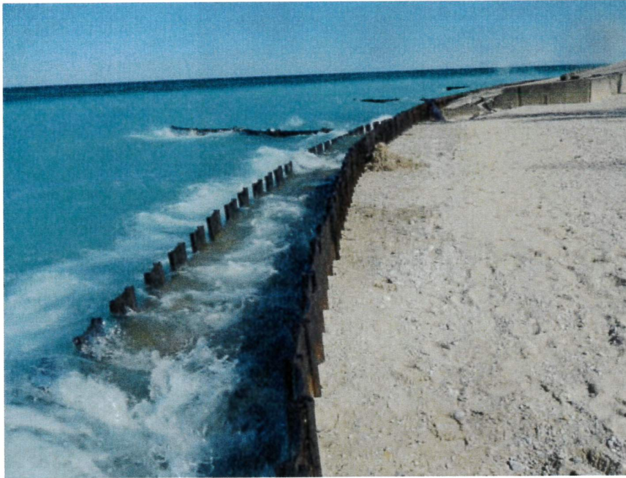
Figure 22: Typical lean in double sheet pile wall (looking north, to the south of the concrete apron). Lean in wall ranged from 4 to in excess of 6 inches.
