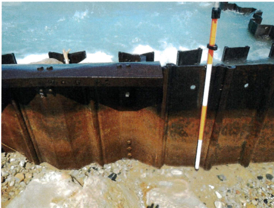
Figure 29: Termination of steel cap beam extending past the north end of the apron. Approximately 3 feet of erosion may have occurred.
