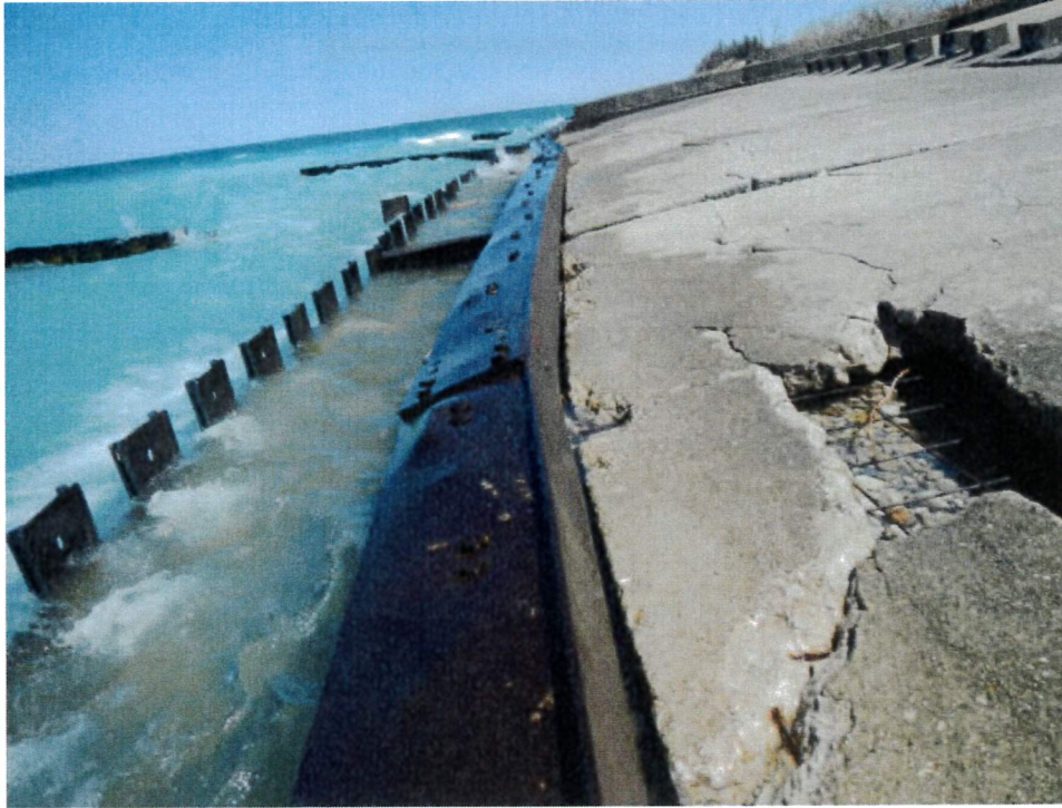
Figure 26: Steel cap beam and double wall (looking north, north apron curb can be observed). Distortion in steel cap beam, lean in wall. Cracking and spalling of apron.
