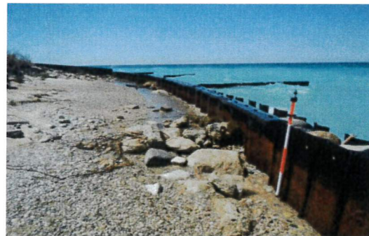
Figure 2.15: Behind double sheet pile wall (looking south, north end of apron can be seen). The 3 feet of erosion extends 20 to 30 ft behind the double sheet pile wall.
