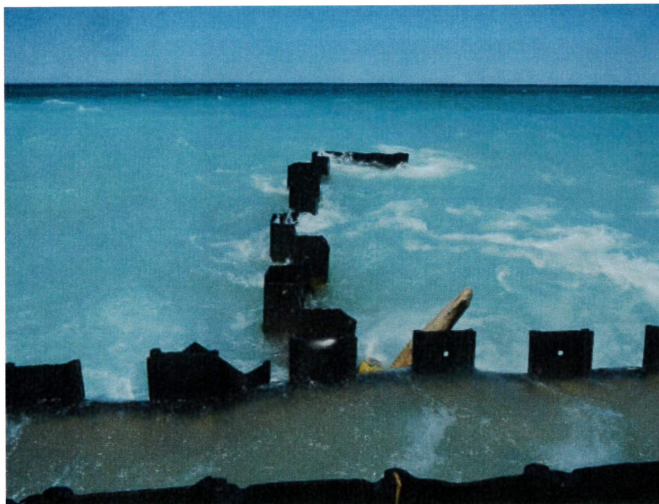
Figure 39: Groin 1 (looking west). Separation between wall and groin. Debris lodged in gap between wall and groin. First sheet pile is either bent or broken.
