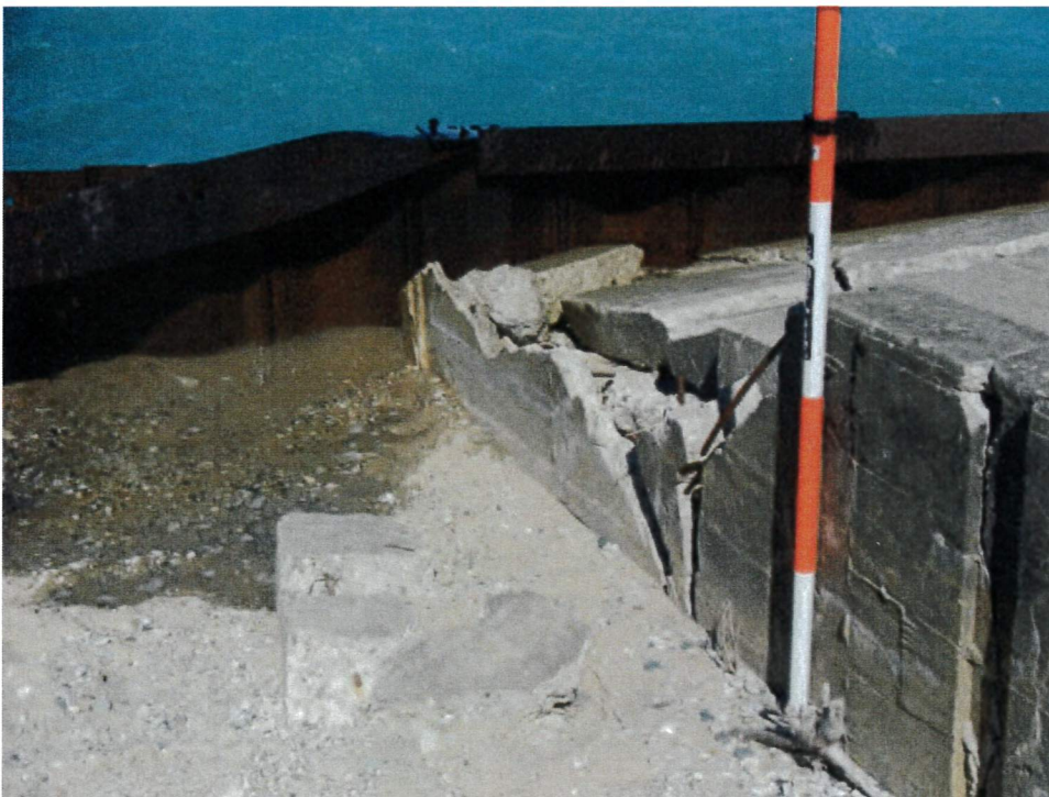
Figure 6: South Concrete Apron (Looking West-Northwest). Apron curb has cracked and settled. Some erosion and washout appears to have occurred to the south of the apron (once the concrete apron ends, extending all along the south extent to the South Return Wall).
