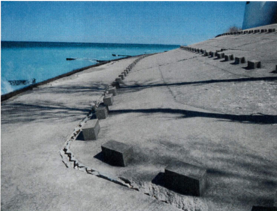
Figure 8: Concrete apron (looking north, near the south end of the apron). Separation between the front 13 feet segment of apron and the back. Exposed steel sheet piling observed within separation. Noticeable change in concrete coloration, and newer cinder block bollards can be seen, indicating the lower 20 feet of apron is newer than the upper portion of the apron.
