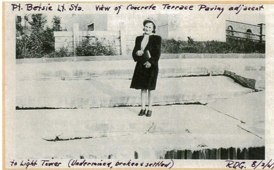
Figure 2.8: Undermining, Breaking and Settling of Concrete Apron, August 1947
