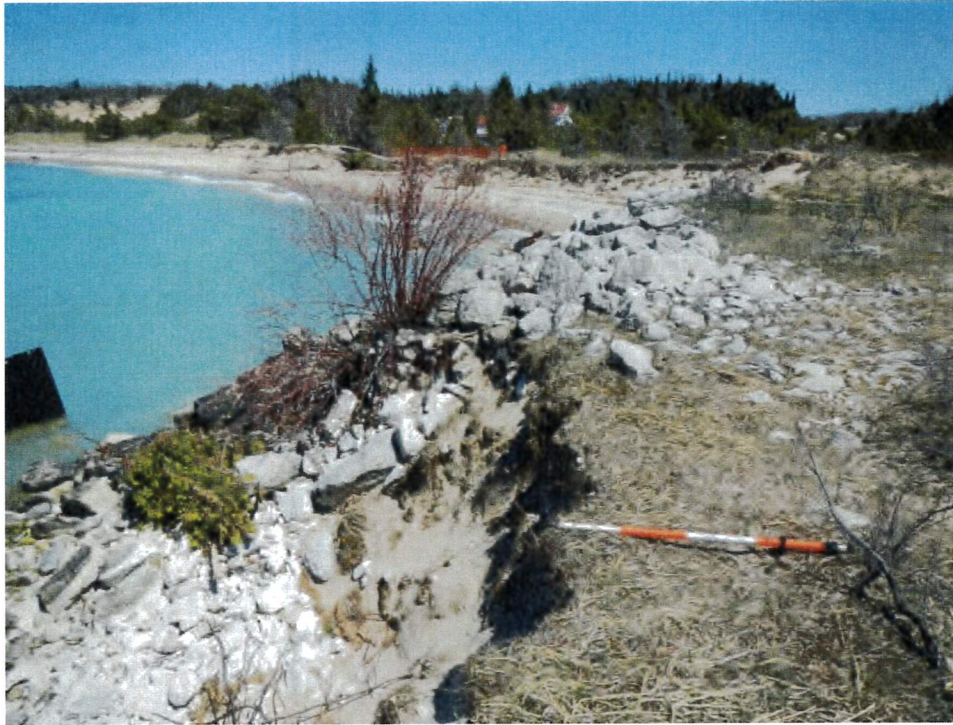
Figure 50: Bluff erosion at west end of stone revetment (looking east). Slope stability failure of bluff, approximately 25 feet wide.
