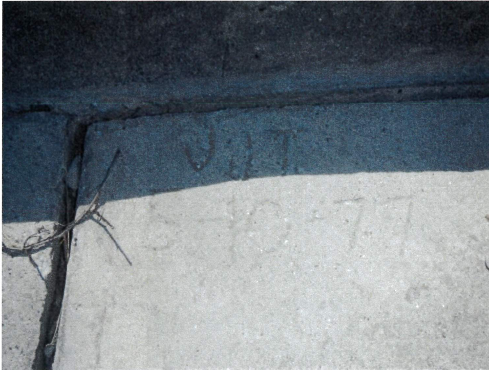
Figure 21: Concrete initials and date (located at southern edge of lower/newer concrete pour, near apron curb). Indicates the lower, and newer, concrete pour was performed in 1977.
