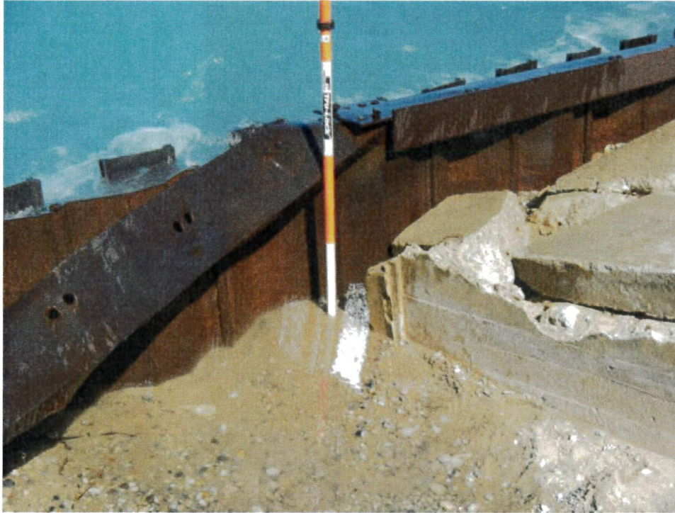
Figure 7: South concrete apron (looking northwest). Settlement in apron. Cracking and spalling. Damage to steel cap beam.
