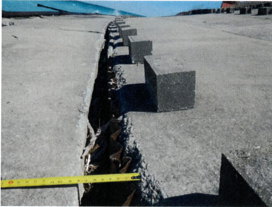
Figure 11: Close view of separation between lower 13 feet segment of apron and the upper portion of apron (looking north)
