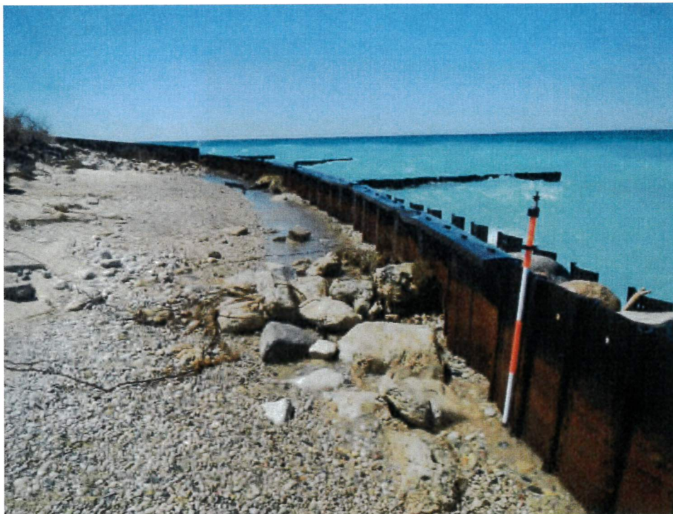
Figure 31: Behind double sheet pile wall (looking south, north end of apron can be seen). The 3 feet of erosion extends 20 to 30 ft behind the double sheet pile wall.
