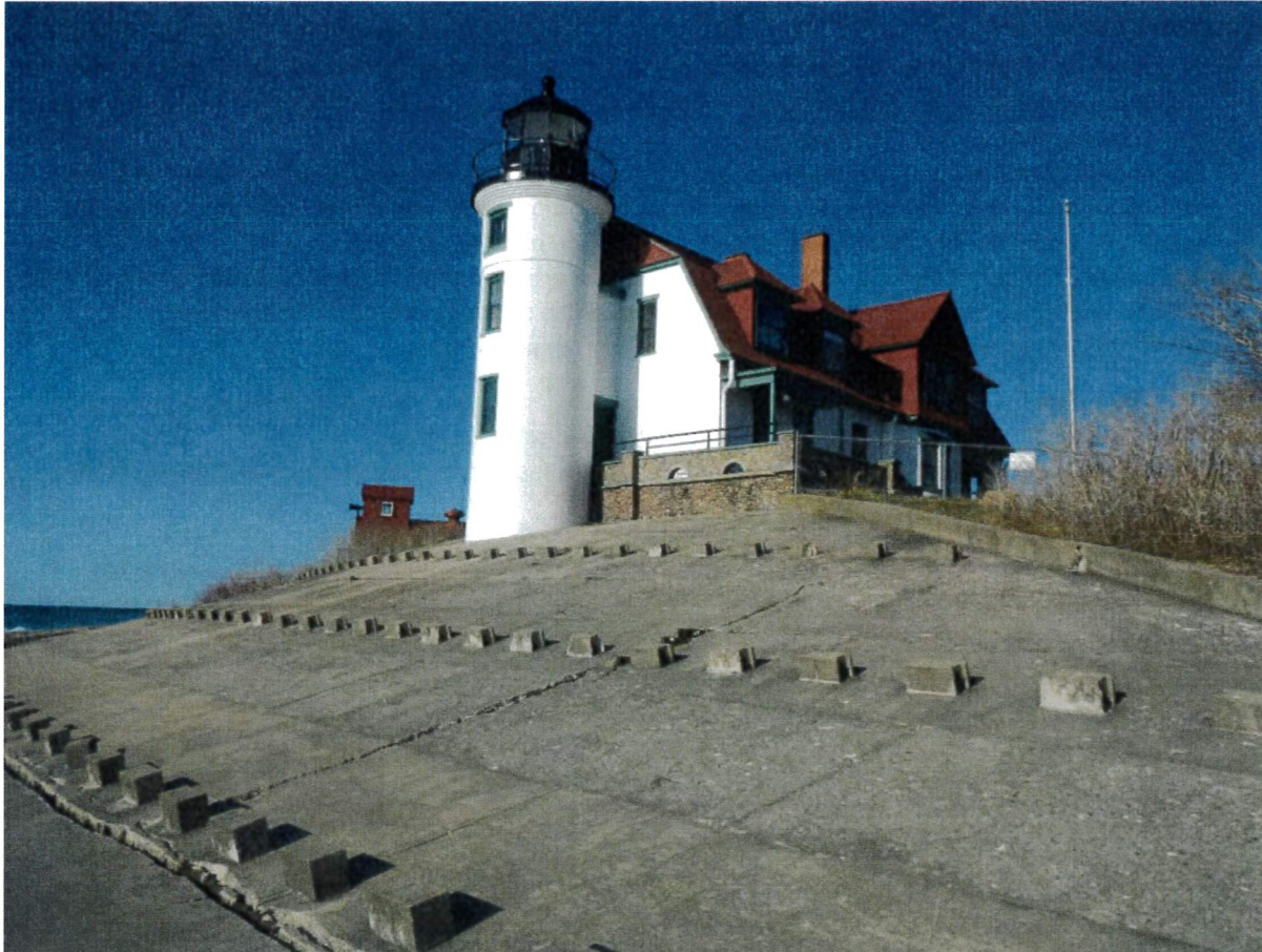
Figure 2: Point Betsie Lighthouse – Concrete Apron and Bollards (looking north from shore)
