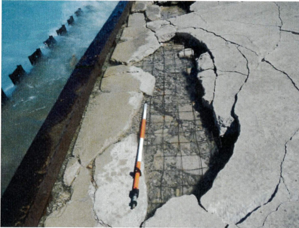
Figure 15: Concrete apron (close up of large cracking and spalled area). Exposed welded wire mesh, mesh does not appear to have been supported during concrete pour, and was pushed to bottom of concrete, where it serves little purpose.
