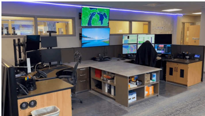
New Benzie County 911 Dispatch Center, March 2024
