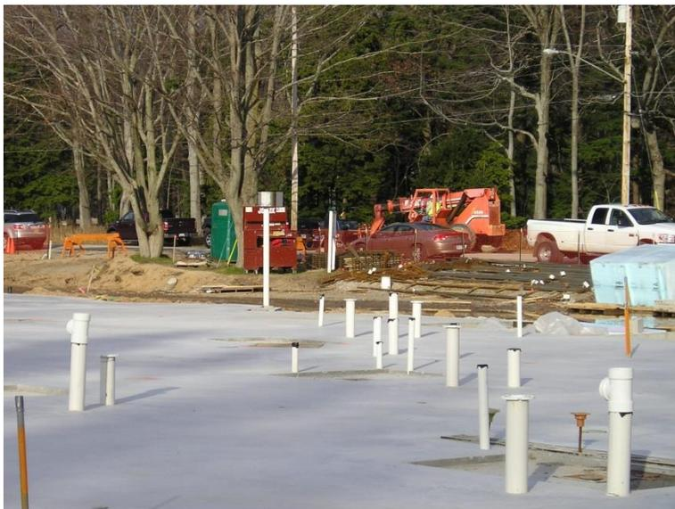
The new entryway foundation slab has been poured.
