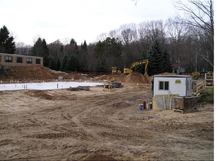
The west module foundation block has been set. Pipe is now in the ground, just waiting on the next load of concrete.
