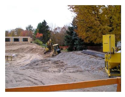
East module foundation set, pipe installed and concrete poured.
