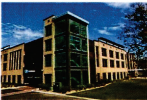
Old Town Parking deck Traverse City, MI May 2011 SILVER CERTIFICATION
