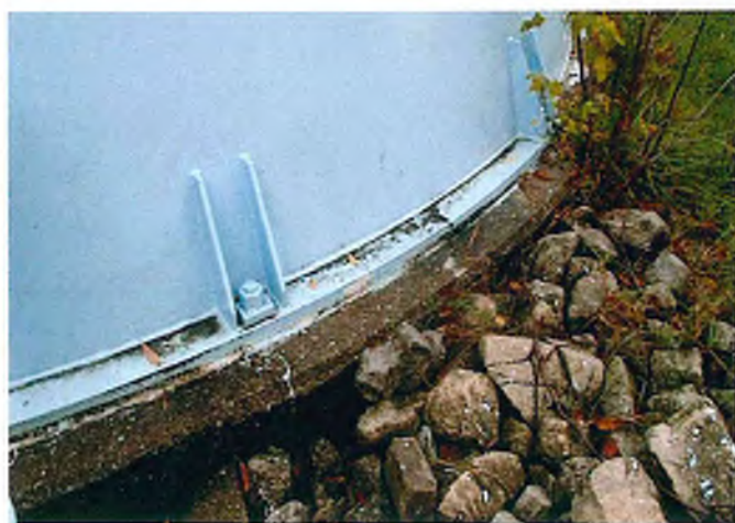
Exterior Base Structure
