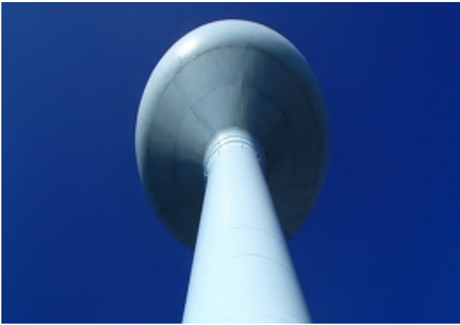
Exterior Coating Pedestal
