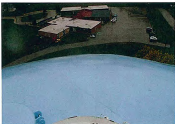
Exterior Coating Roof
