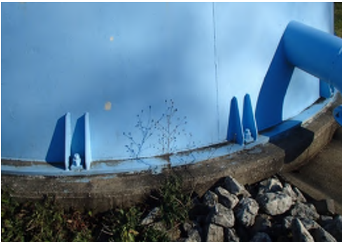
Exterior Base Structure
