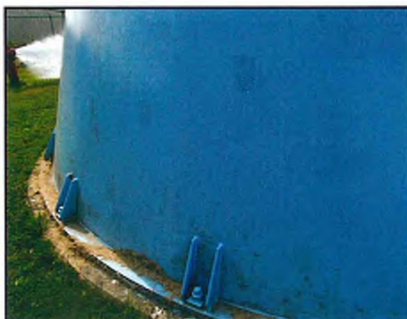
Exterior Foundation and Anchor Bolts
