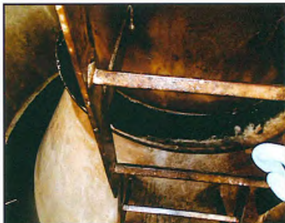
Interior Ladder (Pre-Washout)
