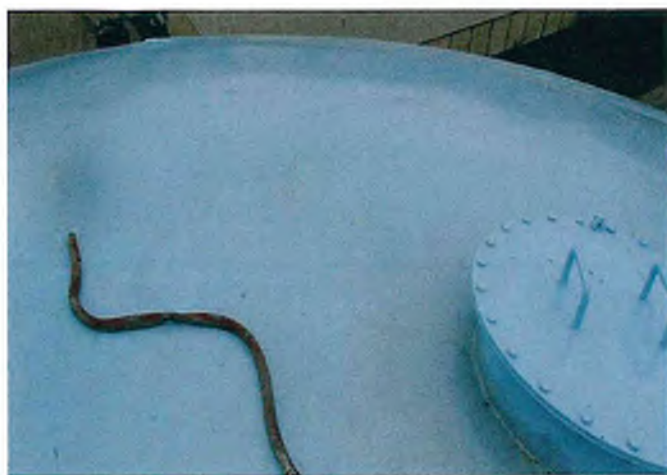
Exterior Roof Structure
