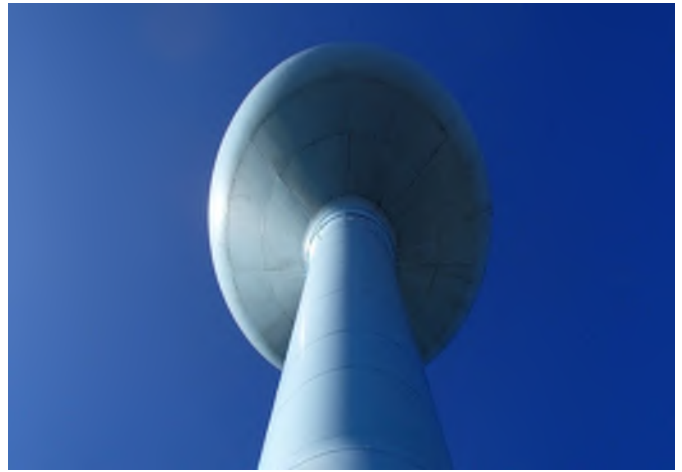
Exterior Coating Pedestal
