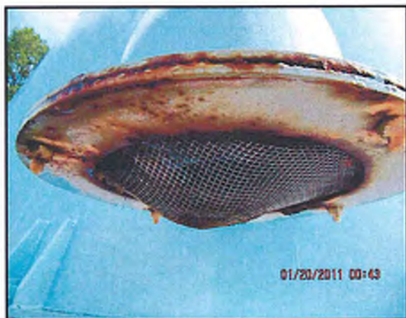
Overflow is equipped with screen.
