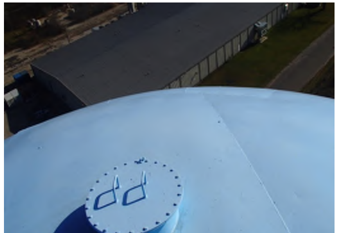
Exterior Coating Roof
