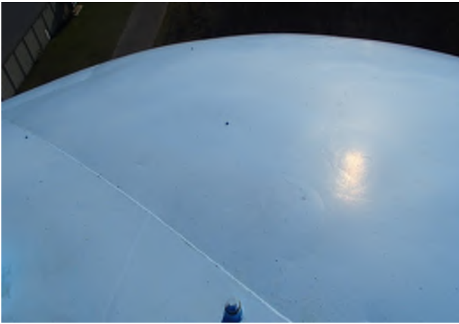
Exterior Coating Roof
