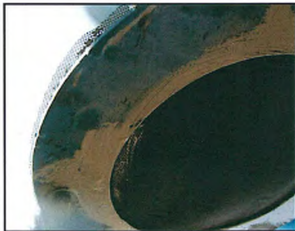
Overflow Screen Replaced
