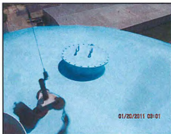
Access hatch is secured.
