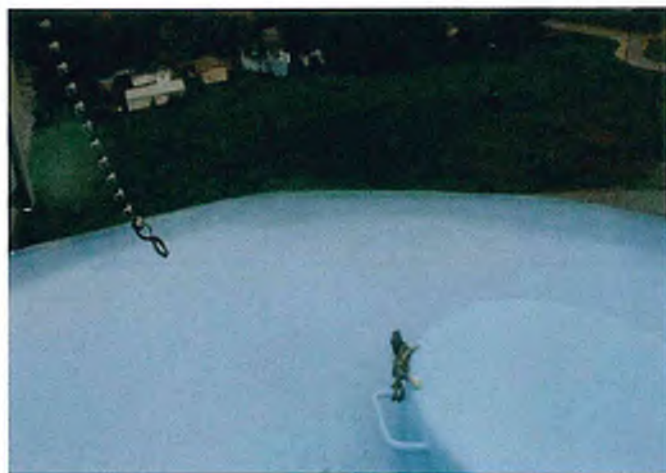
Exterior Coating Roof
