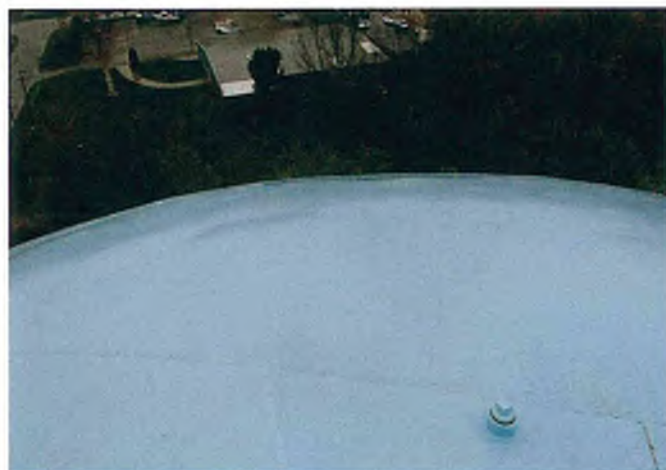
Exterior Coating Roof
