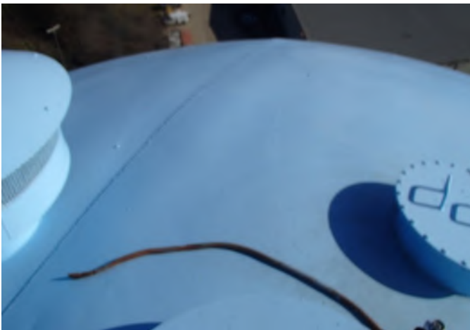
Exterior Coating Roof
