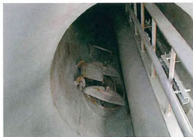
Wet Interior Boiler Manway
