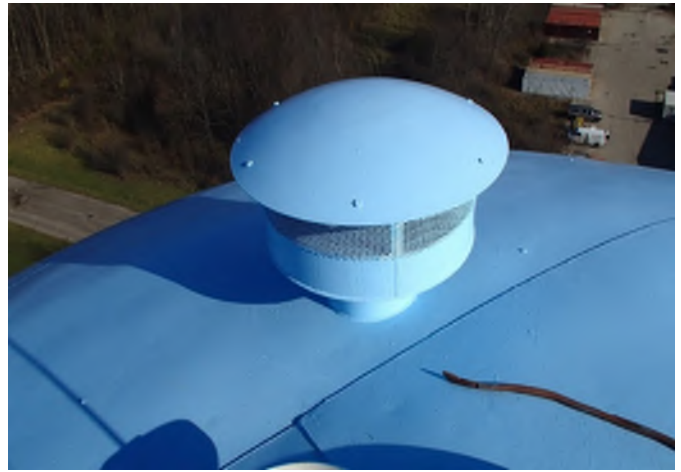
Exterior Coating Roof
