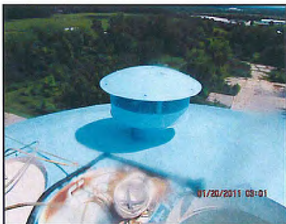
Roof vent is equipped with screen.
