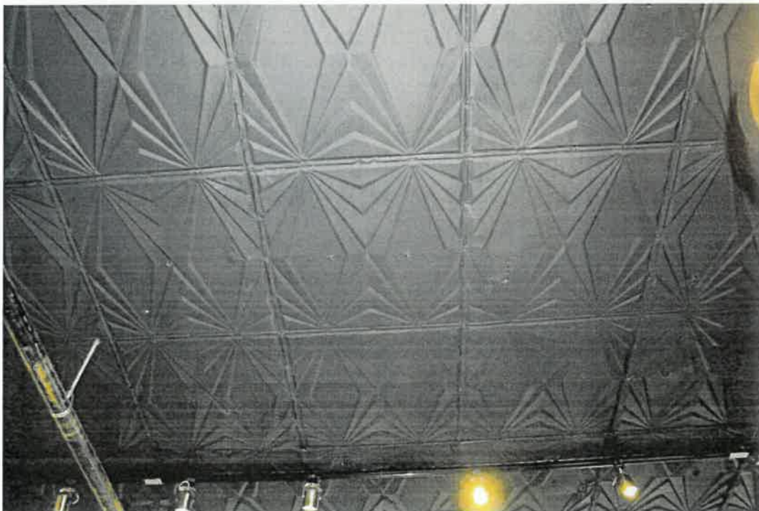
Photo 62 – Restored pressed tin ceiling at first floor commercial space
