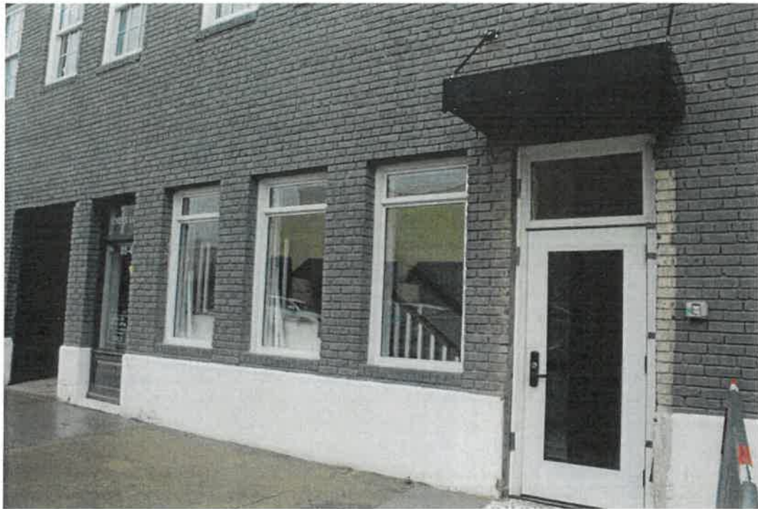
Photo 11 – Restored storefront windows and door, west elevation
