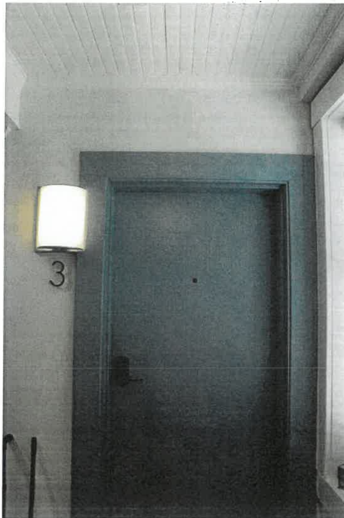
Photo 94 – Flush, fire-rated apartment door
