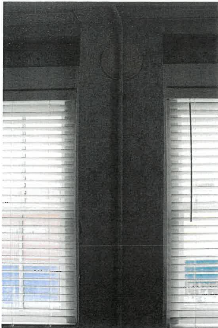
Photo 74 – Restored smooth plaster on south wall
