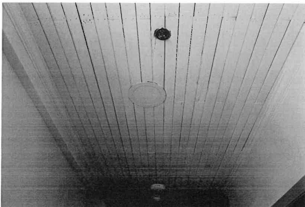
Photo 66 – Beadboard ceiling in second floor corridor
