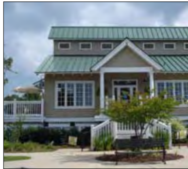
New Riverfront Construction - Conway, 2010
