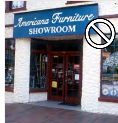
Flat vinyl letters applied to an out-of-scale signboard construction are shown above. The entire sign is set across facade elements such as building piers, banding and slightly over the storefront opening edge. This becomes out of context to the traditional architecture.
