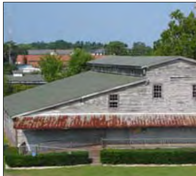
Roofs and rooftop monitors are defining features of historic warehouses. Large expanses of pitched surface is appropriate for metal roofs.
