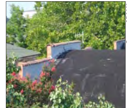
The "fireproof" masonry and barrel vaulted roofs of the warehouses along 2nd Ave, lower, denser "town-side of railroad" forms.
