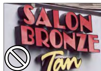
Internally-lit plastic-front channel letters.
