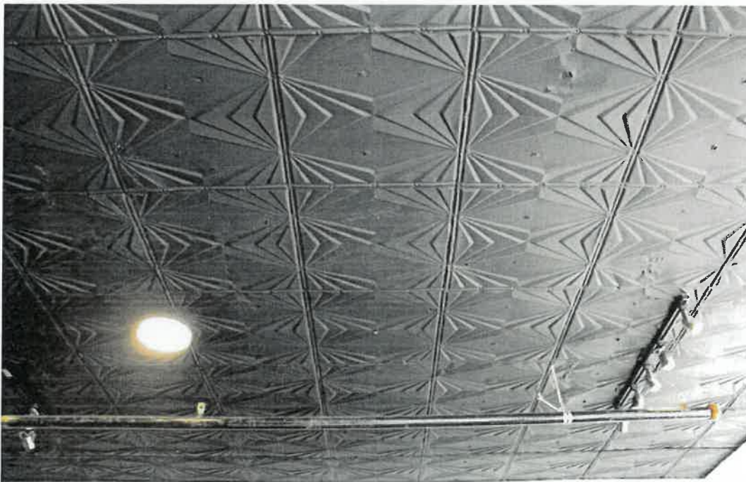
Photo 60 – Restored pressed tin ceiling in first floor commercial block, looking east
