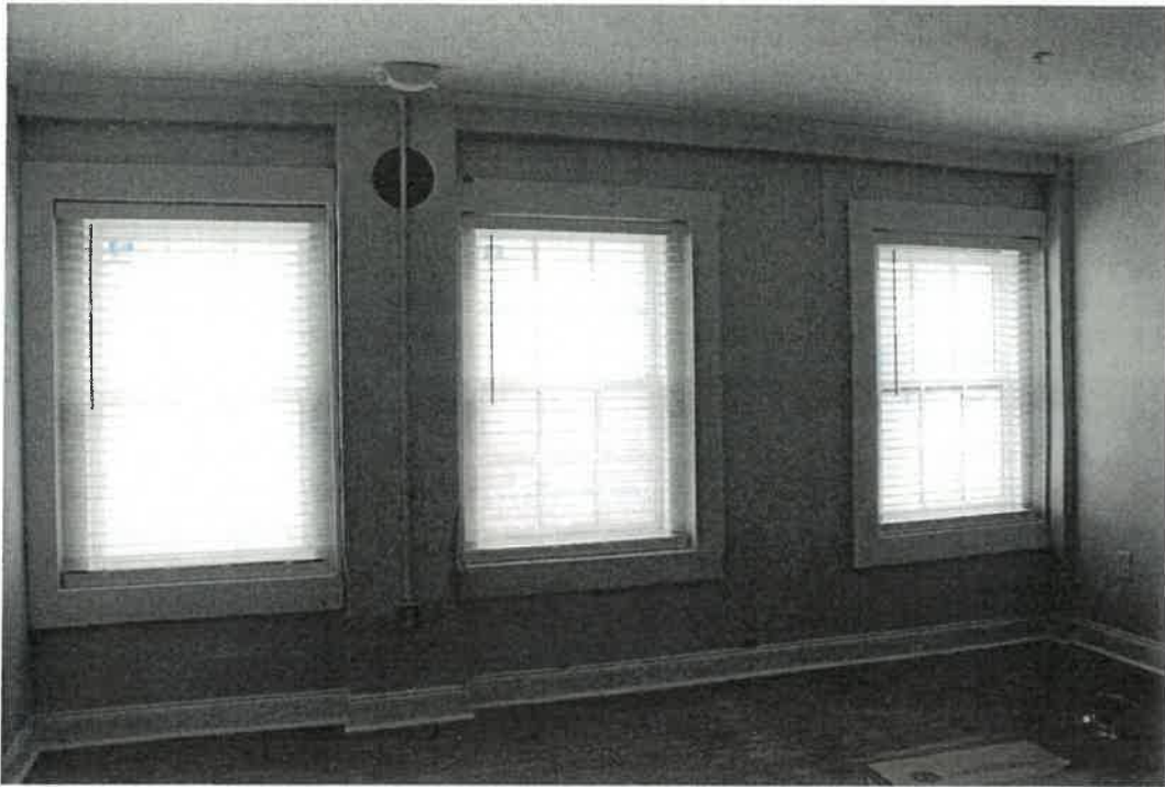
Photo 59 – Restored windows in third floor unit, looking west
