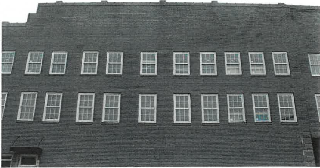
Photo 8 – Restored windows on west elevation
