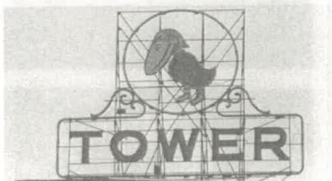
16. (a) The Jayhawk Hotel in Topeka, Kansas, was built in 1926; (b) Its prominent and popular rooftop signs were deteriorating when the hotel closed; (c) The new owners converted the building to offices, but were able to keep the historic signs by changing "HOTEL" to "TOWER." The new, repaired, signs reuse three of the historic letters: T, O, and E. Photos: (a and b) Kiene and Bradley; Courtesy, Kansas State Historical Society; (c) Kansas State Historical Society.
