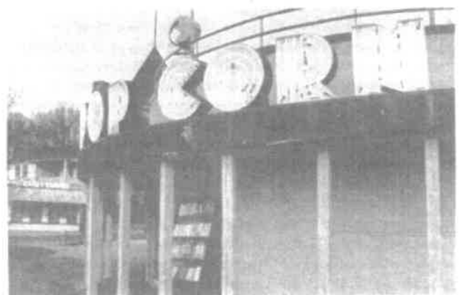
17. Glen Echo Park near Washington, D.C., is an early 20th-century amusement park. (It is the home of the first bumper car ride in the world.) Its neon signs needed repair: (a) tubes were broken and the surrounding "metal cans" needed work also; (b) and (c) removal of the back of "Candy Corner" sign revealed debris from insects and birds; (d) preserving the "metal cans" from the "Popcorn" sign by removing the back; (e) and (f) neon fabricators installing the new tubing in the repaired and remounted cans; (g) repairs finished, the neon signs glow in the park once again. Photos: (a, c) Stan Fowler; (d, f) Larry Kauter; (g) Rebecca Hammer.
