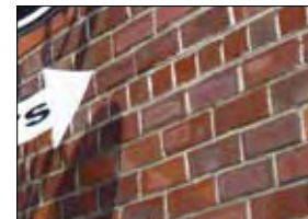
Hand packed or early soft brick w/ soft mortar (ca.1890)
