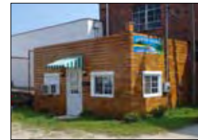
Glazed &amp; high fired brick w/ cast details (1920s-50s)
