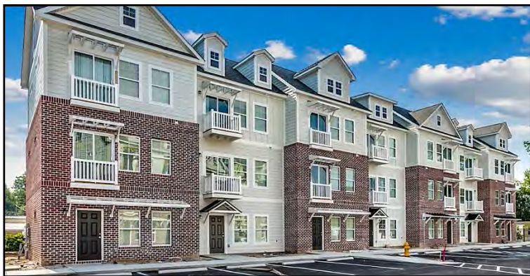
Ex: Brick and Vinyl on all sides (The Wren Coastal Student Housing townhomes)
