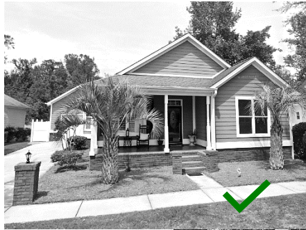
Fig. 2: brick base of same width carried entire length of side of home
