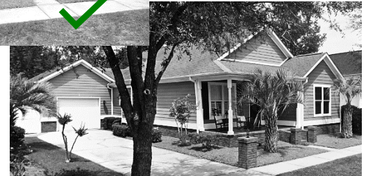
Fig. 2: brick base of same width carried entire length of side of home
