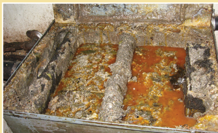
GRD too full of FOG and not maintained properly.
