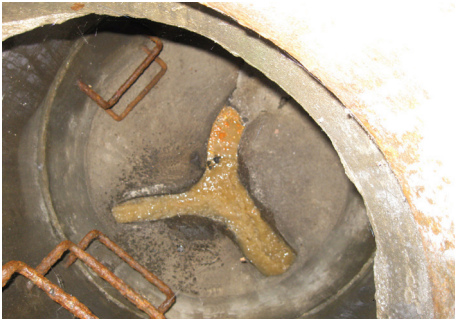
Grease clog in sewer.
