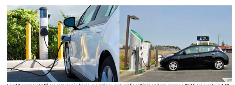
Level 2 chargers (left) are common in home, workplace, and public settings and can charge a BEV from empty in 4-10 hours. Direct current fast chargers (right) are common as public chargers and along highway corridors and can charge a BEV to 80 percent in under an hour. (123RF and <u>Washington State Department of Transportation</u> photos)
