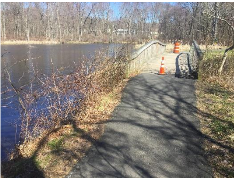
REPAIRS AT MURIEL HEPNER PARK
