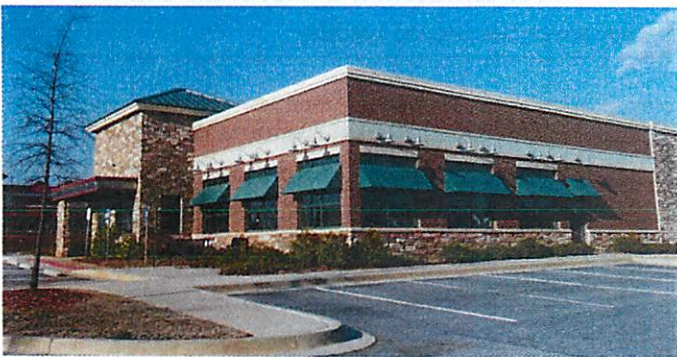
Example of a highly-visible customer entrance with accompanying landscape.
