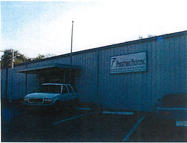
Example of prohibited material
