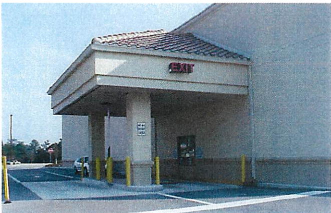
Example of unacceptable drive-through The photo shows an Unacceptable example; the structure needs to extend over the entire width of the second drive-through lane.
