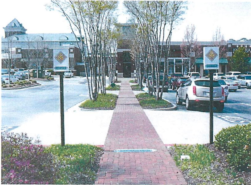
Example of pedestrian walkway and crosswalk The concrete and colored brick pavers effectively identify this pedestrian crossing, increasing pedestrian safety and visibility.
