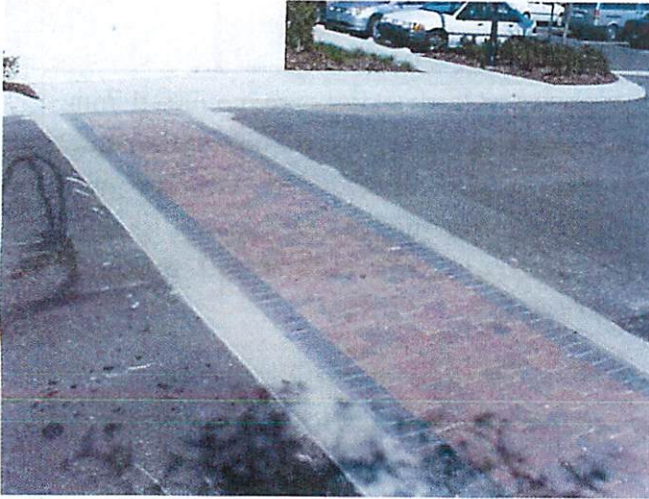
Example of pedestrian walkway and crosswalk The concrete and colored brick pavers effectively identify this pedestrian crossing, increasing pedestrian safety and visibility.
