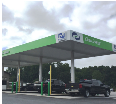
Clean energy station Doraville
