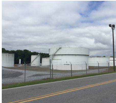
Tank farm Doraville
