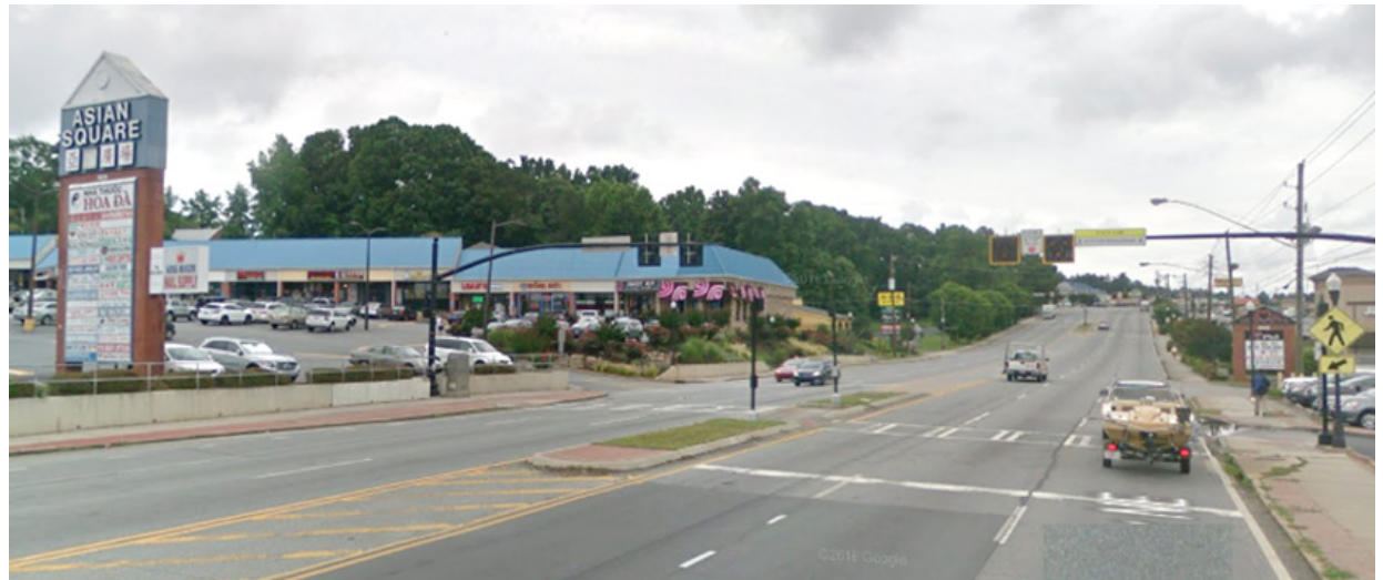
Installation of mid-block crosswalks and HAWK signals (High-Intensity Activated Crosswalk Beacons) along Buford Highway have increased pedestrian safety where installed. Additional transportation and pedestrian safety improvements on Buford Highway will be developed during the Buford Highway Livable Centers Initiative (LCI) Study.
