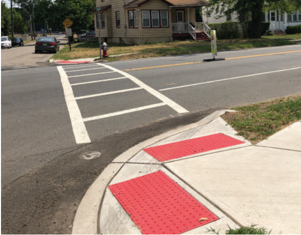
CURB RAMP RECONSTRUCTION
