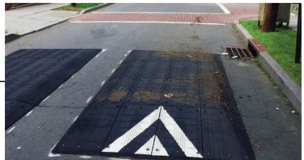
SPEED CUSHION Example of a portable speed cushion that can be anchored temporarily to test its effectiveness.
