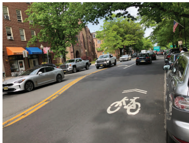
SHARED LANE MARKING
