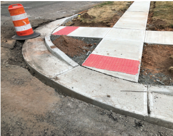
SIDEWALK, CURB, AND CURB RAMP RECONSTRUCTION
