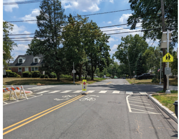
CROSSWALK VISIBILITY ENHANCEMENTS
