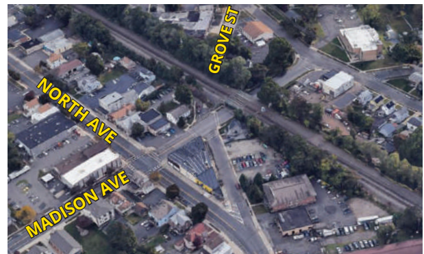
AERIAL IMAGE OF THE RARITAN VALLEY LINE EMBANKMENT WITH A GRADE-SEPARATED CROSSING AT MADISON AVENUE
