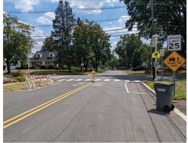
CROSSWALK VISIBILITY ENHANCEMENTS
