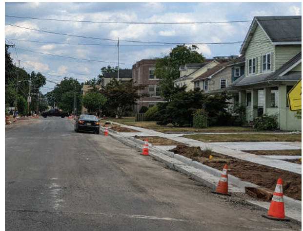
CONTINUE SIDEWALK REPAIR AND REPLACEMENT
