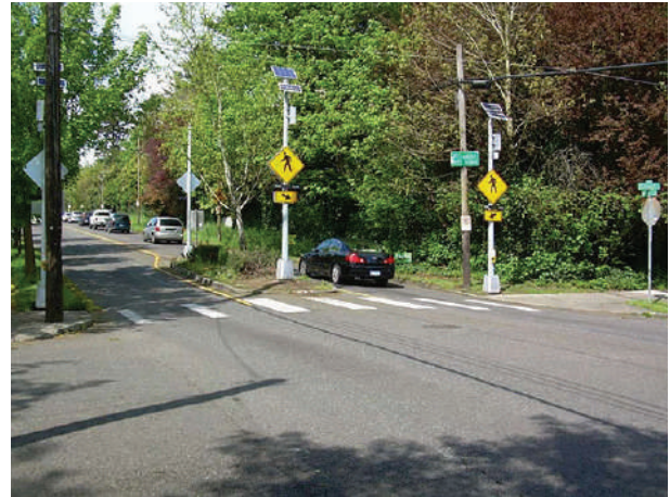
MEDIAN ISLAND WITH INTEGRATED RRFB
