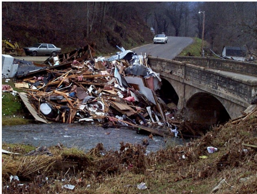
Figure 4-2. Damage from 1998 Flood Event.
