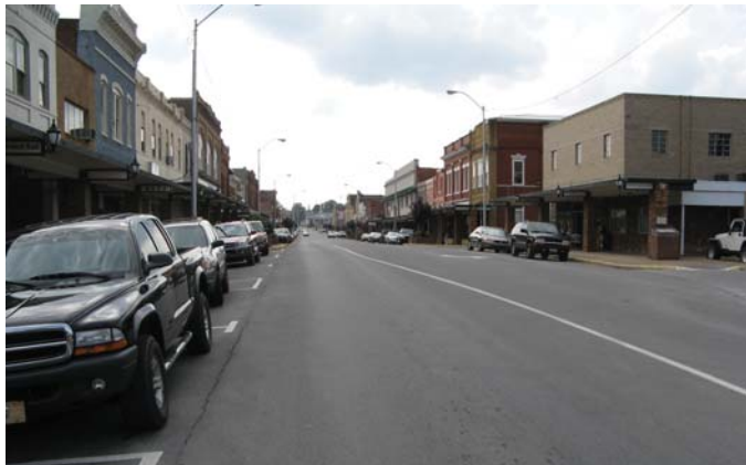
Project M-2. Elizabethton's Downtown Enhancement Plan provides guidance on returning Elk Avenue to two-way traffic. Bike lanes should also be considered downtown. A downtown circulation study would validate the Enhancement Plan findings with technical analysis.
