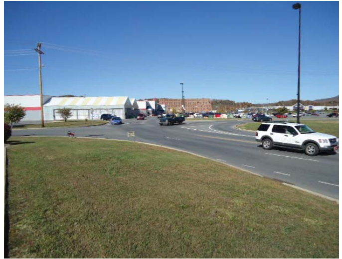
Project S-7. Several options, from simple restriping to complete intersection reconstruction exist to mitigate inefficient operations at the intersection of Hudson Drive and Over Mountain Drive.
