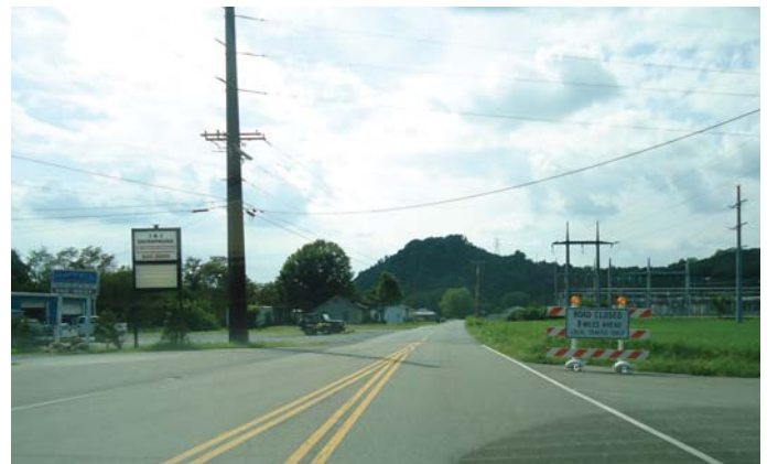
Project M-5. SR 91 east drops its state route designation and narrows to a two lane roadway at SR 37. Its alignment continues as Lovers Lane along the river to SR 400..
