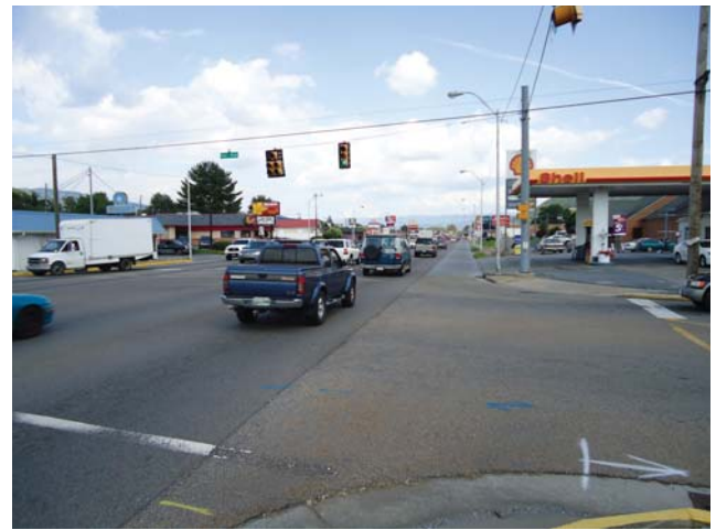
Congestion on Broad Street, on the US 321 corridor. At least one objective of projects M-5, L-1, L-2, L-3, and L-4 is to alleviate growing congestion here.
