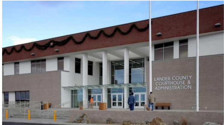
Lander County Courthouse & Administration Building Source: Eleventhjudicialdistrict.com , 2015
