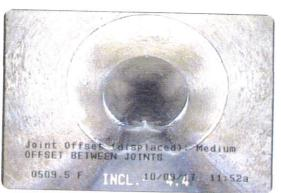
Joint Offset (displaced): Medium at 509.5 feet | OFFSET BETWEEN JOINTS
