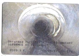
Deformed Vertically at 109.3 feet, 5% (diameter) | DEFORMED AT LATERAL
