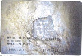
Hole in Pipe: Void Visible at 091.0 feet, 9 o'clock, 1 in | HOLE IN PIPE
