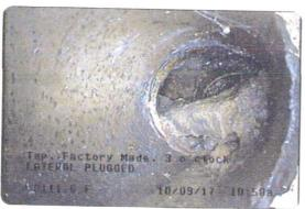
Tap, Factory Made at 111.6 feet, 3 o'clock, 4 in | LATERAL PLUGGED
