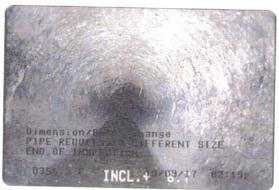
Dimension/Shape Change at 355.3 feet, 4 in | PIPE REDUCES TO DIFFERENT SIZE END OF INSPECTION
