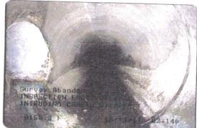
Survey Abandoned at 158.9 feet | INSPECTION ENDS LATERRAL INTRUDING CAMERA STOPPED
