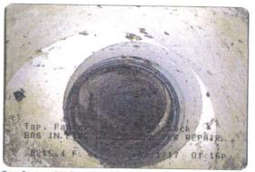
Tap, Factory Made at 215.4 feet, 9 o'clock, 4 in | SAG IN PIPE AT LATERAL PER REPAIR
