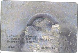
Survey Abandoned at 341.1 feet | PLUGGED AFTER SECOND FLUSH INSPECTION ENDS
