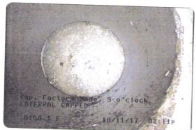
Tap, Factory Made at 150.1 feet, 9 o'clock, 4 in | LATERRAL CAPPED
