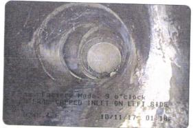
Tap, Factory Made at 246.4 feet, 9 o'clock, 4 in | LATERAL CAPPED INLET ON LEFT SIDE
