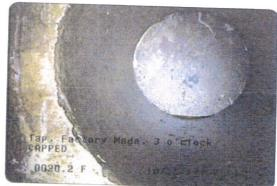
Tap, Factory Made at 020.2 feet, 3 o'clock, 4 in | CAPPED
