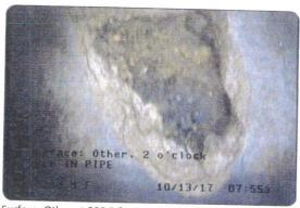
Surface: Other at 298.9 feet, 2 o'clock | HOLE IN PIPE
