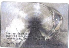
Survey Abandoned at 108.4 feet | INSPECTION ENDS AT LATERAL CONTRUDING BLOCKING CAMERA
