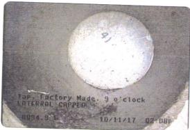
Tap, Factory Made at 094.9 feet, 9 o'clock, 4 in | LATERRAL CAPPED
