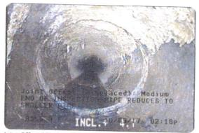
Joint Offset (displaced): Medium at 355.3 feet | END OF INSPECTION PIPE REDUCES TO SMALLER PIPE
