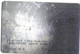
Fracture Longitudinal at 316.0 feet, 9 o'clock, 0 in | LONGINTUDE CRACK DOWN PIPE
