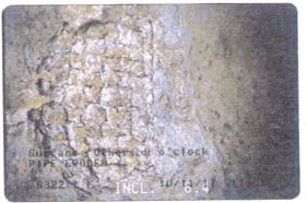
Surface: Other at 322.1 feet, 9 o'clock | PIPE ERODED
