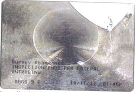
Survey Abandoned at 066.9 feet | INSPECTION ENDS PER LATERAL INTRUDING
