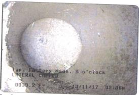
Tap, Factory Made at 039.2 feet, 9 o'clock, 4 in | LATERAL CAPPED
