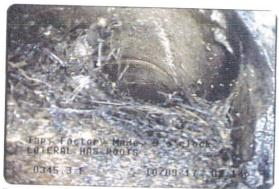
Tap, Factory Made at 345.0 feet, 9 o'clock, 4 in | LATERAL HAS ROOTS
