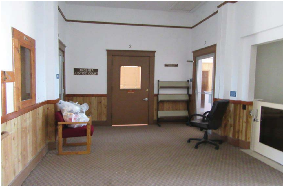
Photo 6. Lobby on first floor. Historic fabric shown includes the doors and frames, baseboard, wainscot, and picture rail. The paneling appears to be later.
