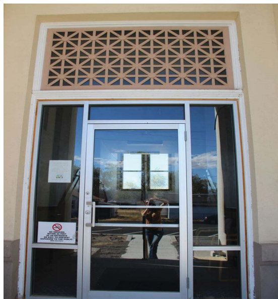
Photo 4. Aluminum storefront door. Not original. The recommendation is to remove this assembly and replace it with an entry that matches the original design.
