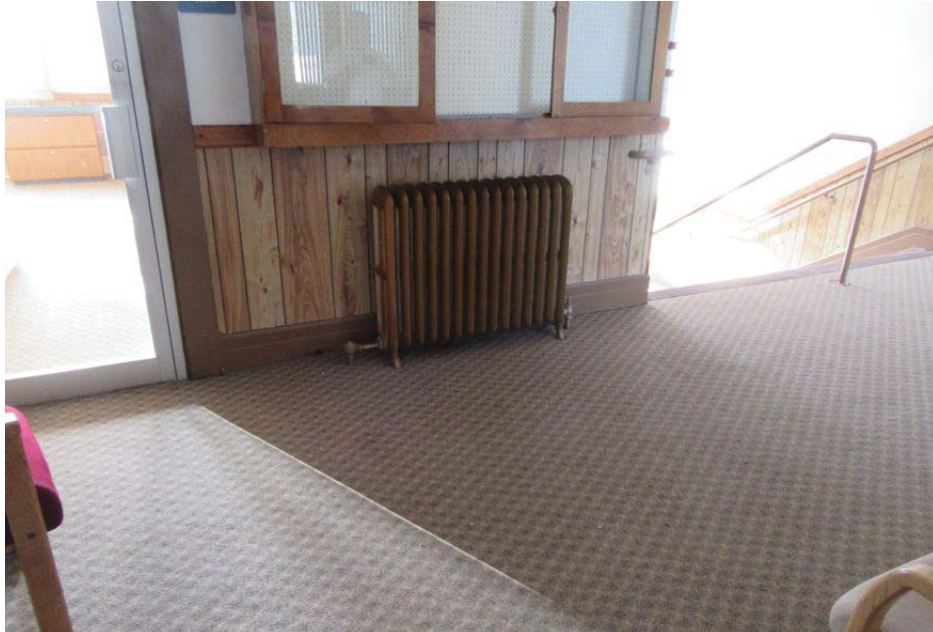
Photo 8. Interior of first floor lobby. Radiators are an important element of the historic fabric, even though they are not functional. The aluminum door to the left should be replaced with a wood door matching the others in the building.
