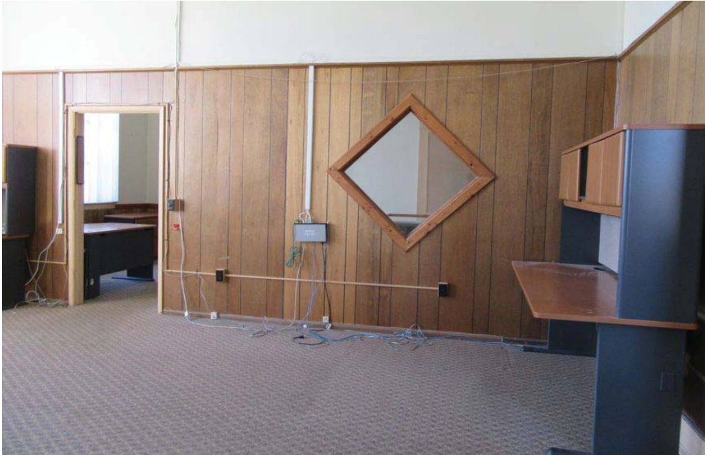
Photo 7. Interior walls, and wall finishes, constructed for the Courthouse use are removable and the plaster and flooring patched.
