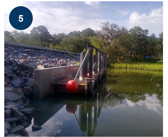
Figure 5.12 - 5.14 Bottom, Left to Right). Precedent imagery of stormwater wetlands, wet enhanced swales, and muted tide gate.
