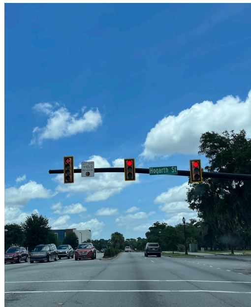
Figure F.5 Flashing yellow arrow and new signal heads on Boundary Street in Beaufort.
