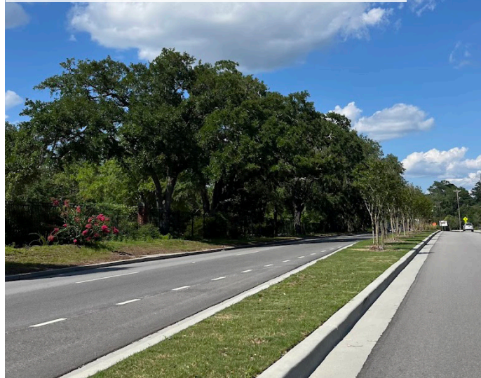
Figure F.7 Example of raised and landscaped median in Walterboro on S Jefferies Boulevard. This project was completed in 2023 and the medians replaced a center two-way left-turn lane.
