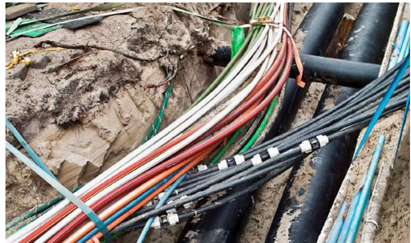
Electrical and communication lines are bundled and buried
