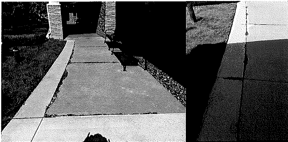
Colored Concrete Sidewalk Spalling in Front of Library
