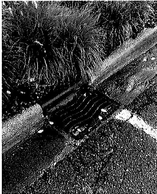
Inlet Filter Remaining in Catch Basin
