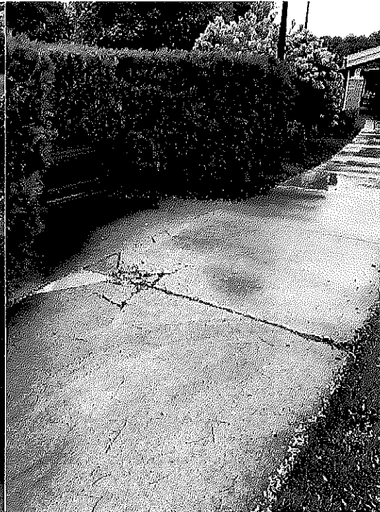
Spalling NE Corner of South Lot
