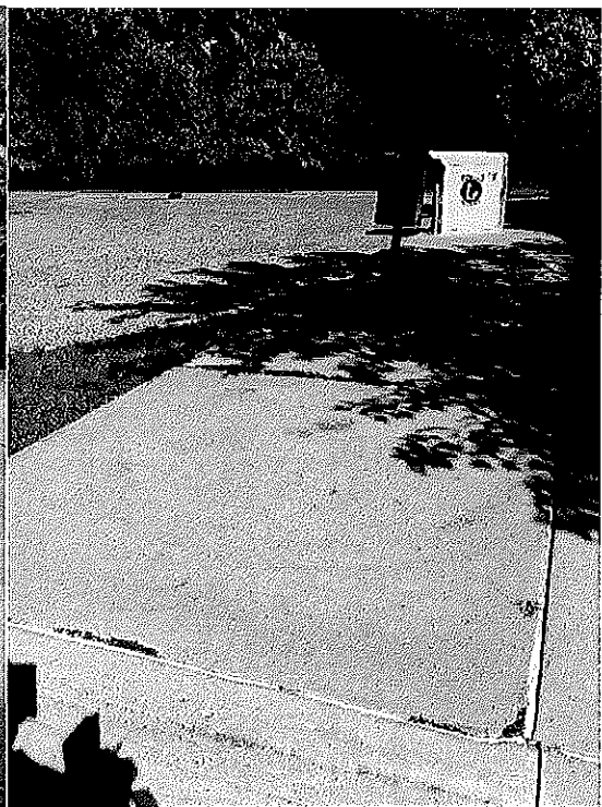
Spalling Sidewalk N of Bldg.
