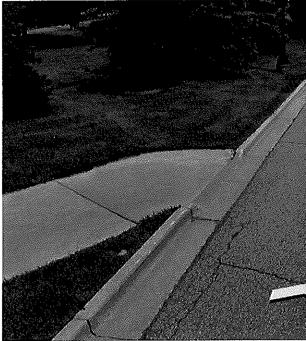
Sidewalk Cracking North End of North Lot
