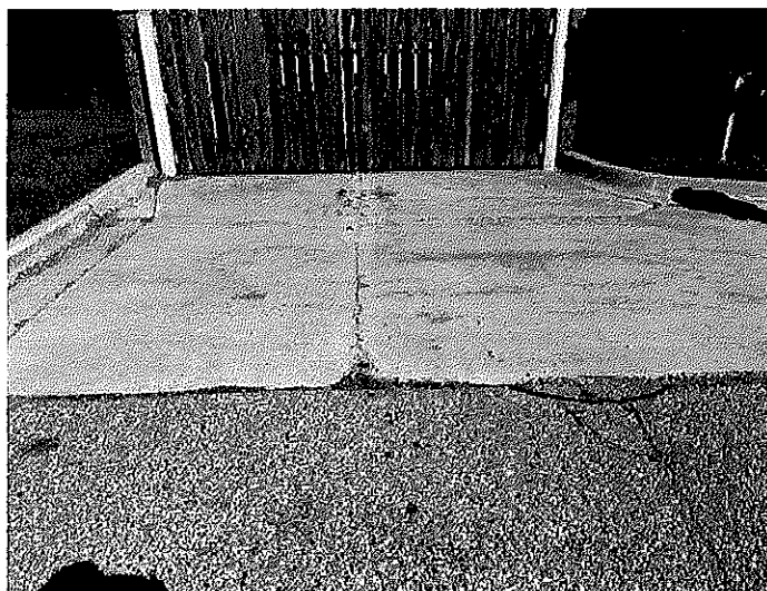
Concrete Spalling at Dumpster Pad
