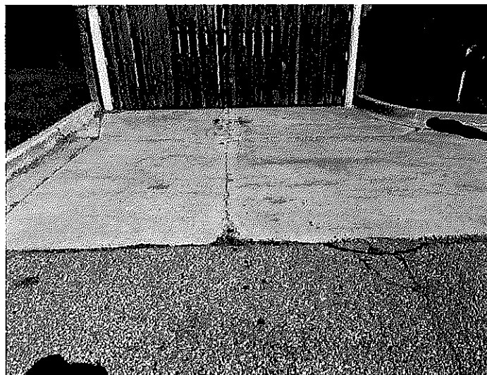
Concrete Spalling at Dumpster Pad
