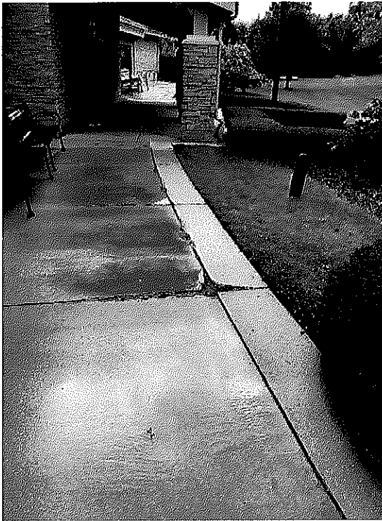
Colored Concrete Spalling
