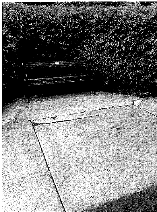
Cracking/Spalling Near N Bench Bldg. Entrance
