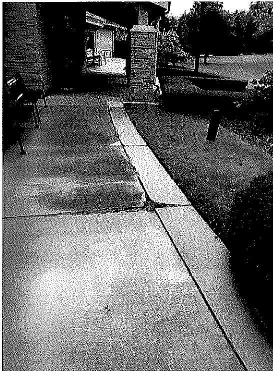
Colored Concrete Spalling
