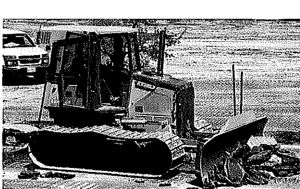
Example of Dozer Removing Asphalt
