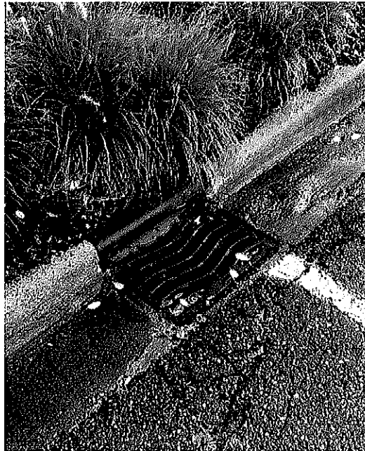
Inlet Filter Remaining in Catch Basin
