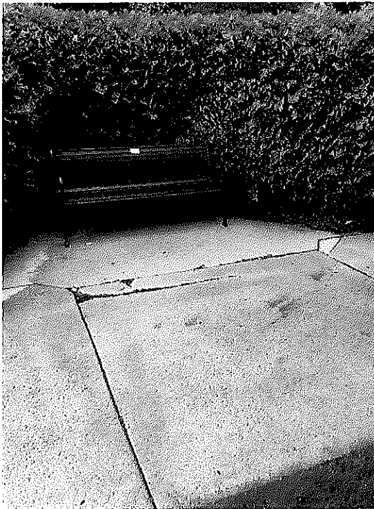
Cracking/Spalling Near N Bench Bldg. Entrance
