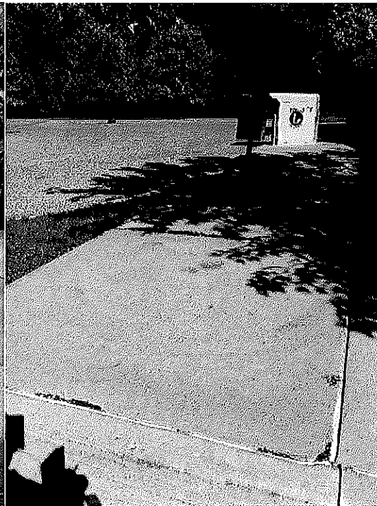
Spalling Sidewalk N of Bldg.
