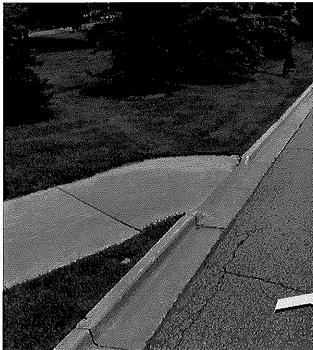
Sidewalk Cracking North End of North Lot
