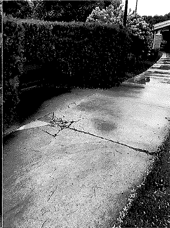
Spalling NE Corner of South Lot
