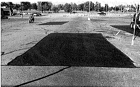
Asphalt Patching and Crack Sealing Example
