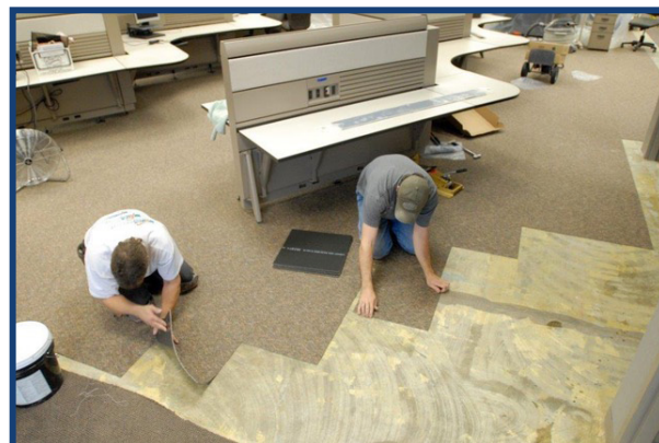
The field carpet is installed.
