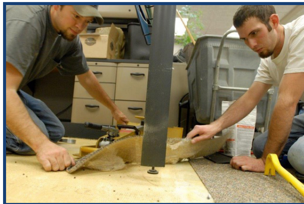
We gently pry up the partitions to facilitate old carpet removal.
