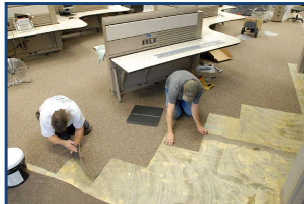
The field carpet is installed.
