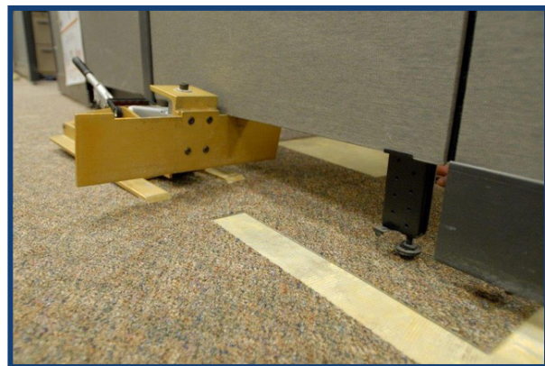
Mini-lift equipment is inserted under work stations, and we slide new carpet tile underneath.
