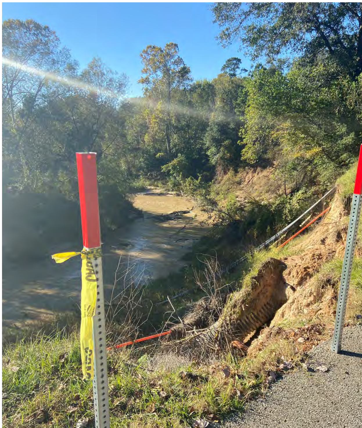
Stewart Creek vegetative debris within channel and erosion at Magnolia Drive (guardrail, gas line, and stormwater pipes have collapsed with bank
