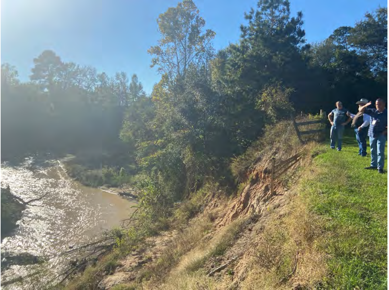
Streambank failure at residence/yard located north of proposed improvements
