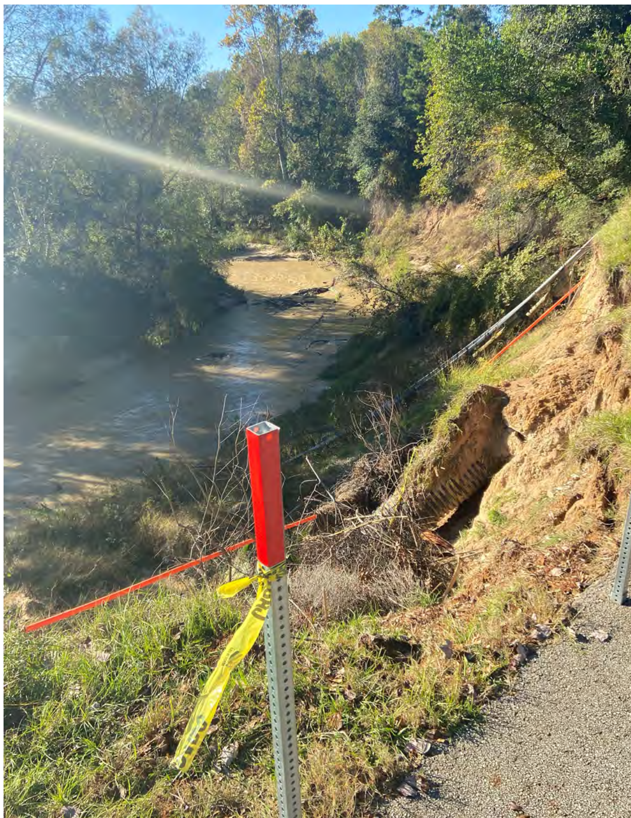
Stewart Creek vegetative debris within channel and erosion at Magnolia Drive (guardrail, gas line, and stormwater pipes have collapsed with bank
