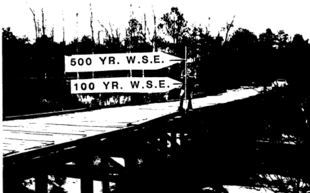
Figure 2. – Potential flood heights at Sycamore Drive over Caney Creek.
