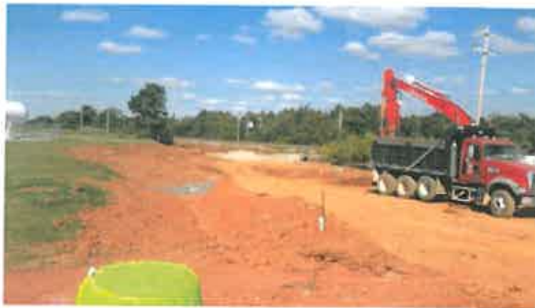
Photos of Overexcavated Area after being backfilled
