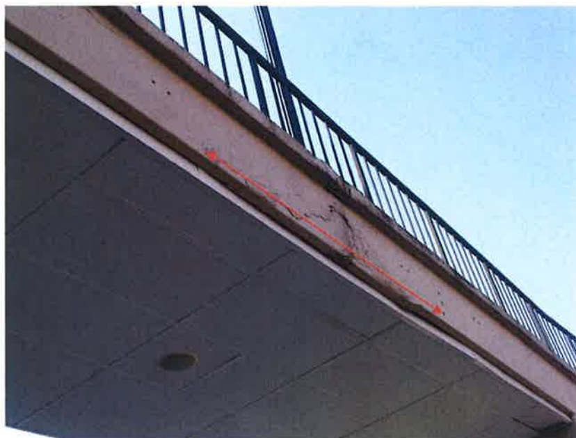
COLLISION DAMAGE TO BEAM "A" AT APPROACH #1 (NOTE: BEAM BROKEN) (NOTE: COVERED W/ PANELS 2019)
