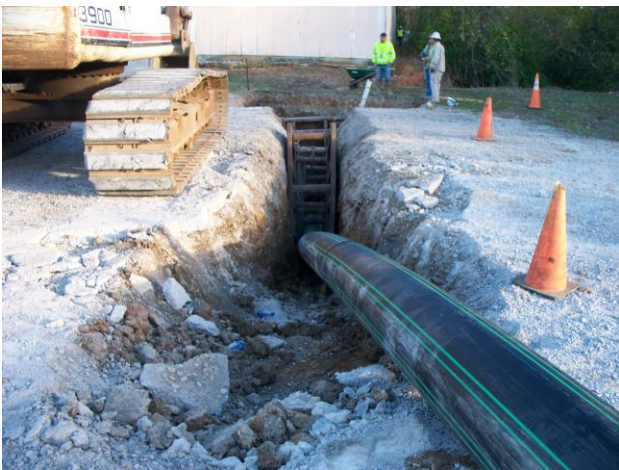
Directional Bore Under Building
